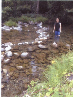
Repairing wingdam at POD for ditch irrigation July 7, 2016 at 5:25:44 PM
