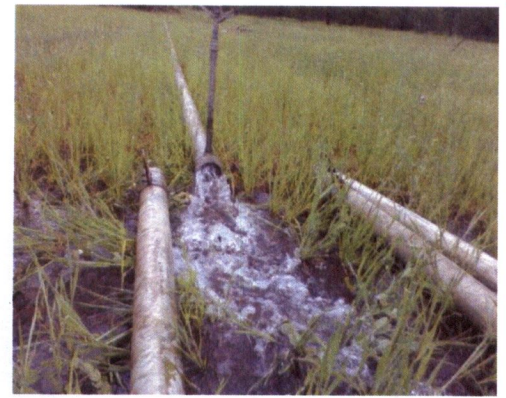
Flushing out sprinkler pipe near middle of WR May 17, 2013 at 11:19:23 PM
