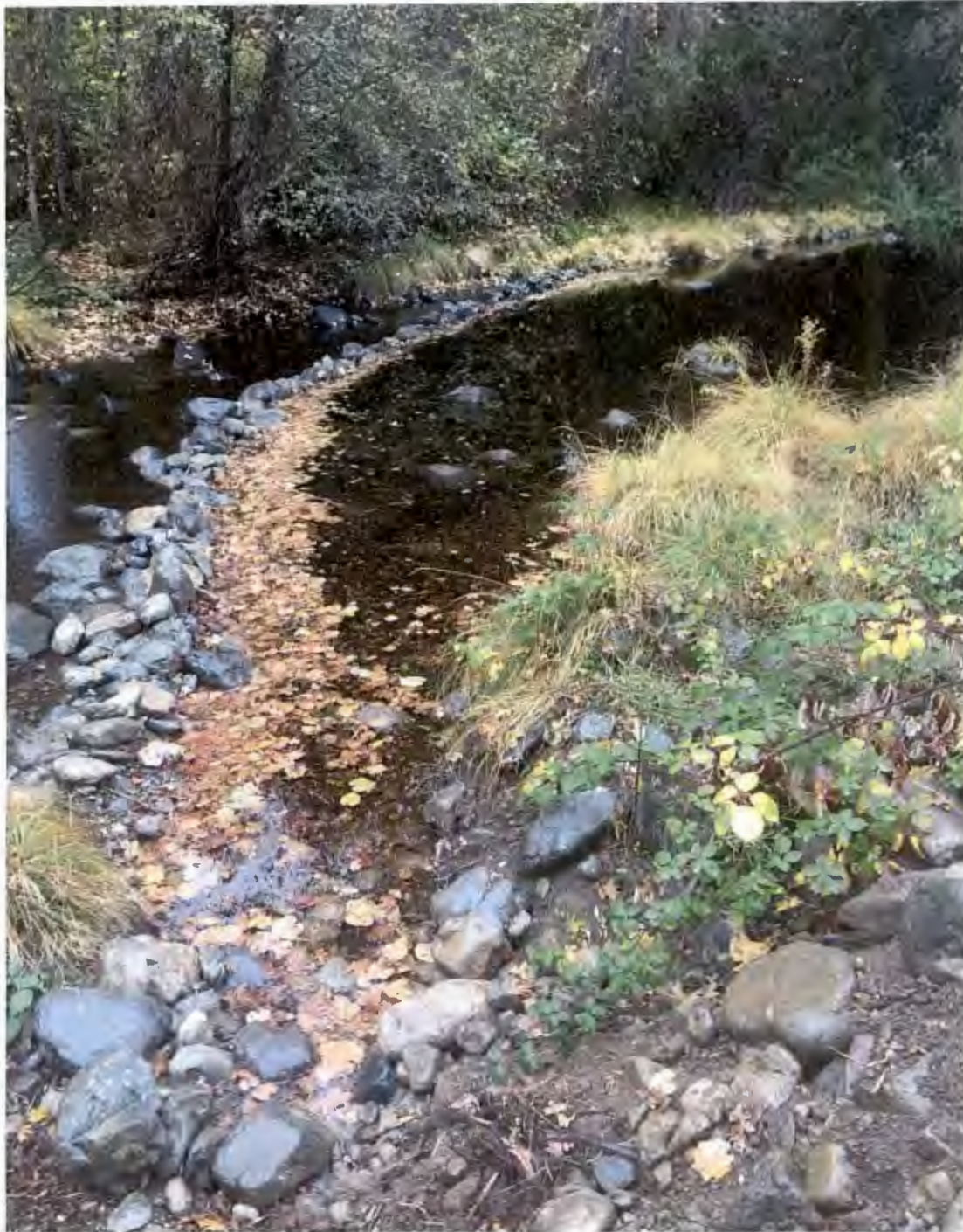
Photo 1 – Existing diversion location showing remnant cobbles from pushup dam. Potential passage barrier during low flows.
