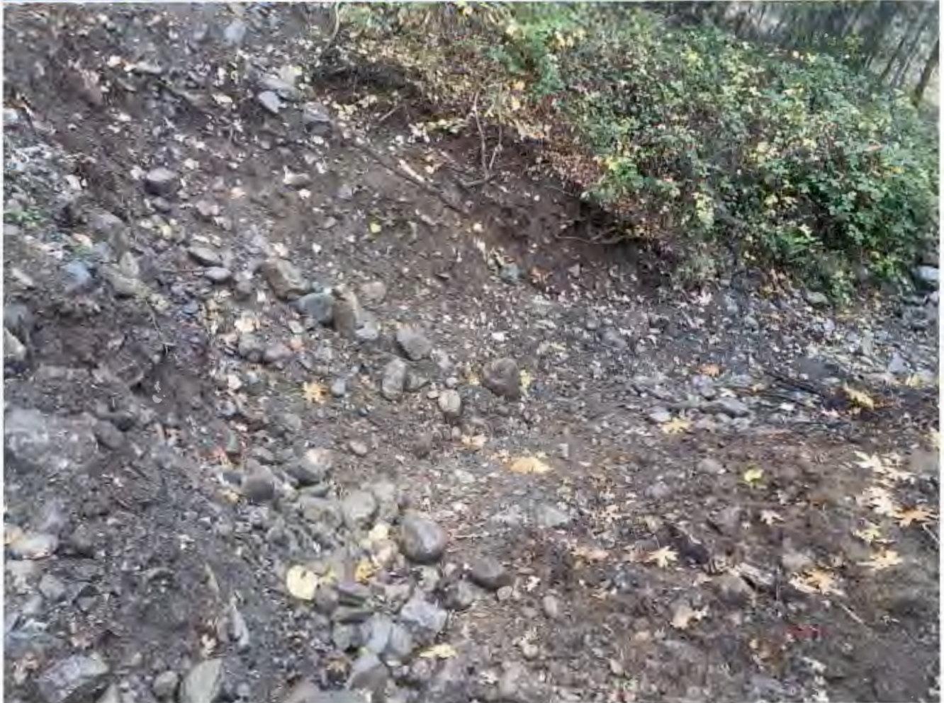
Photo 2 – Existing diversion channel and potential stranding hazard located south of the pushup dam location. Notice the non-native blackberry and lack of vegetation within the riparian area.
