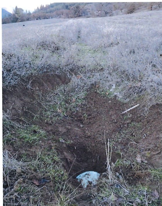
Figure 6: End of 10" pipe section, entering open ditch on North East field.
