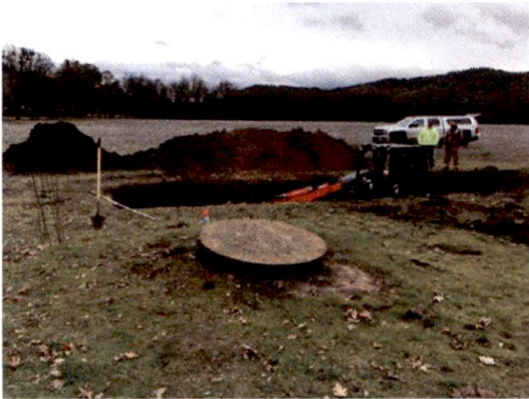
3. Test location relative to 1953 Dug Sump.
