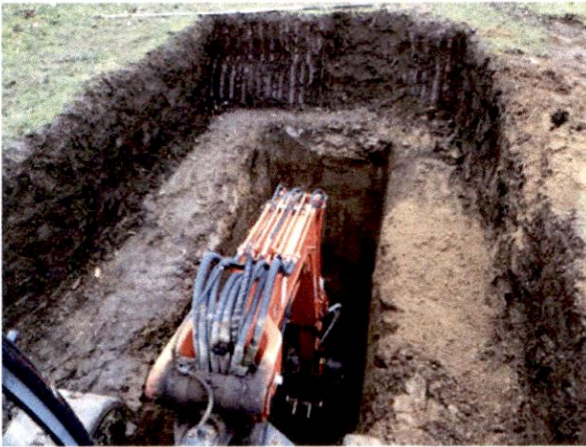
1. Test Pit Excavation.
