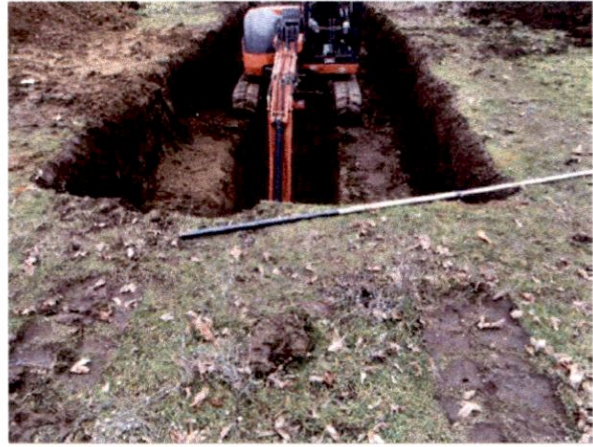
4. Test Pit Excavation.
