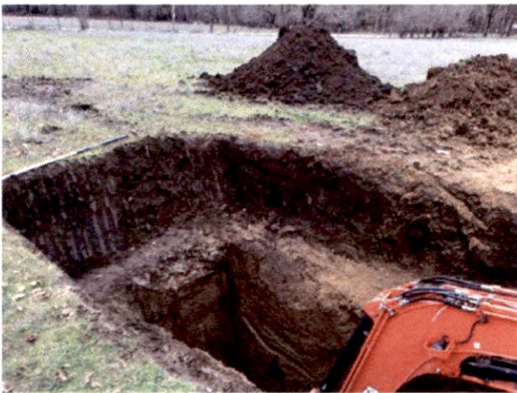
2. Test Pit Excavation with separate piles of different lithologies.
