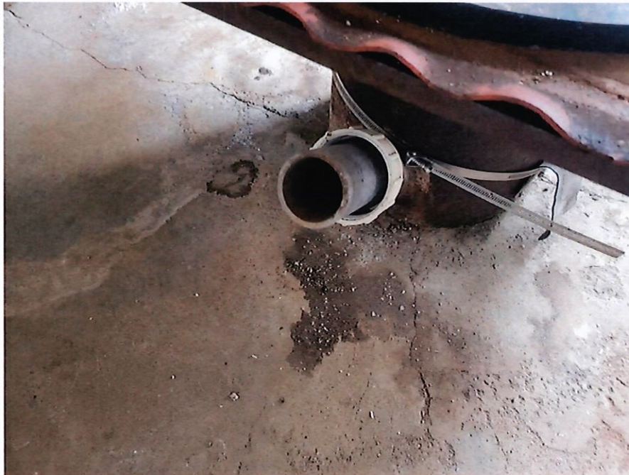
Well #3 Access Port
