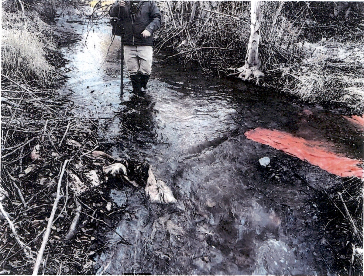
The photo above was taken on 1-19-21 and shows water being diverted through the Bear Creek Diversion.
