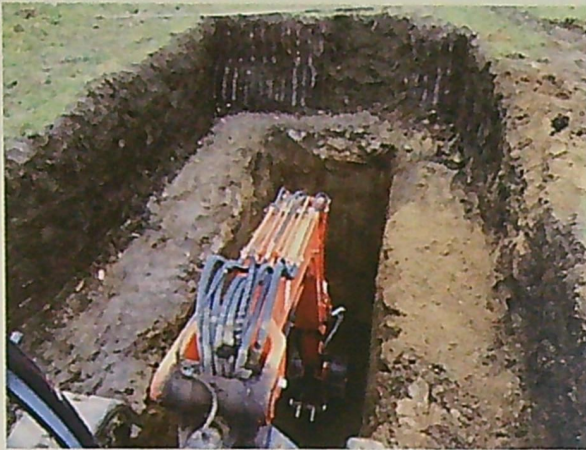
1. Test Pit Excavation.
