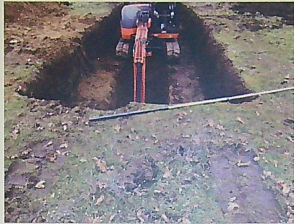
4. Test Pit Excavation.
