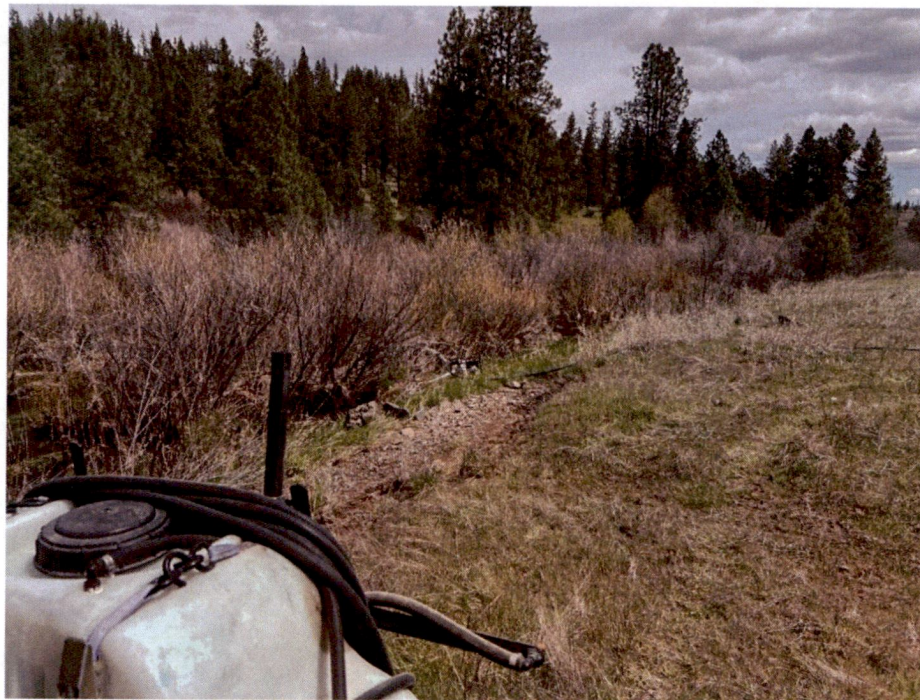
Figure 20: POD 10 with pump station in operation
