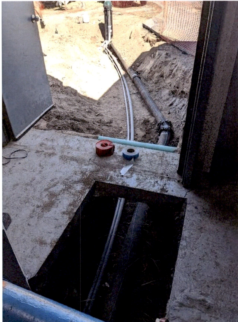
Photograph 2. The above photograph shows the piping from the new pitless unit well head into the building and tie-in to the existing water system. The piping is ductile iron water pipe with MegaLug flanges, NSF 61 approved materials.
