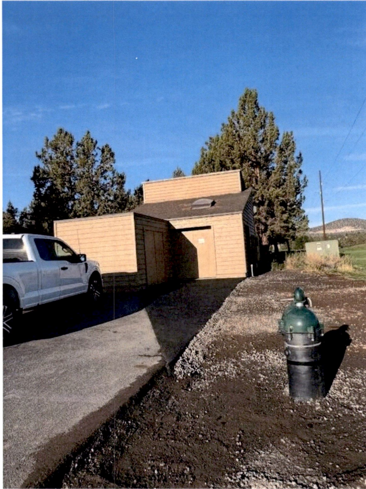
Photograph 3. The above photograph shows the completed well head with pitless unit (with integrated sampling port) with the previous Photograph 2 pipe trench completed and asphalt patched for building approach for maintenance equipment access.
