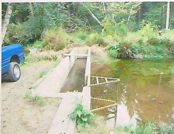
Fish ladder at bottom of spawning pond, no flash boards in place.
