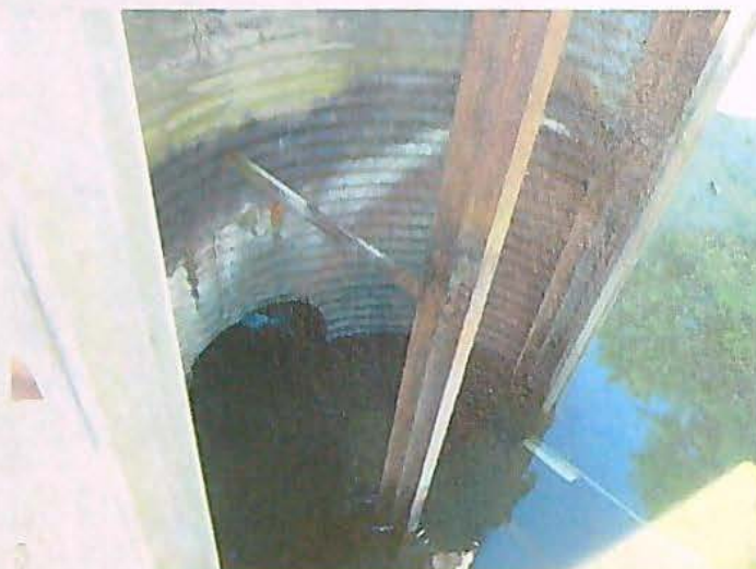
Rearing pond outlet structure. No flash boards in place at this time.
