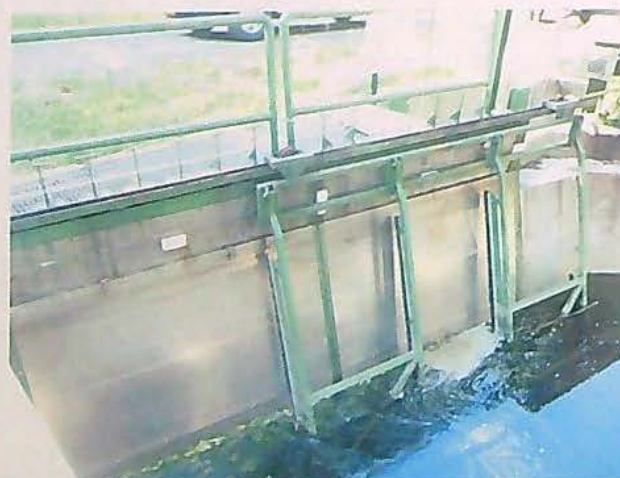
Fish screen and by-pass structure.
