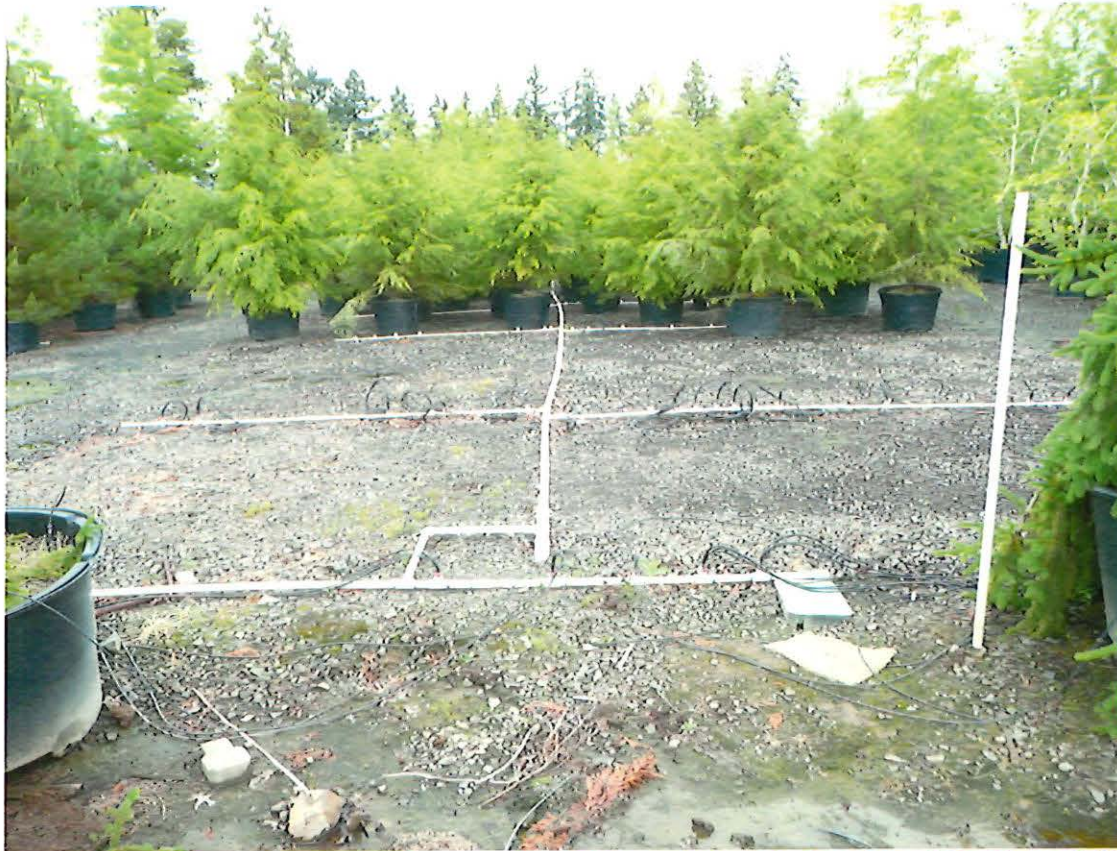
One portion of the sales yard using pvc hand line and drip irrigation, drip lines visible.
