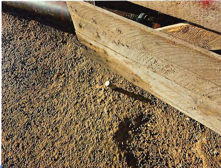
Well #7 Access Port
