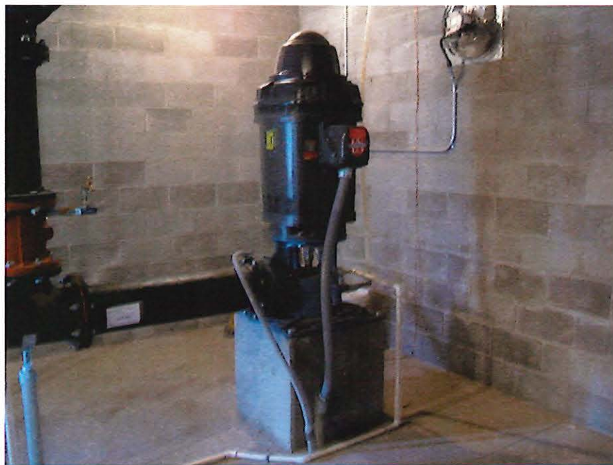
PUMP AND MOTOR ASSEMBLY
