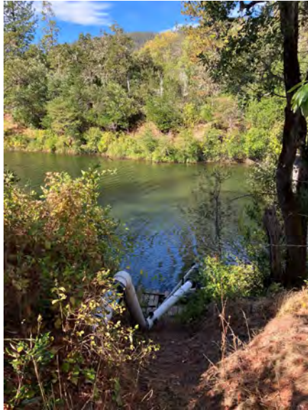
Figure 3. Sweet Cron Farm pump in Illinois River at POD (9/2024).
