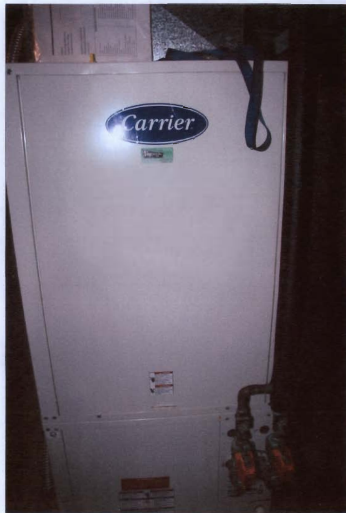
Above - Carrier heat pump 2-26-2008
