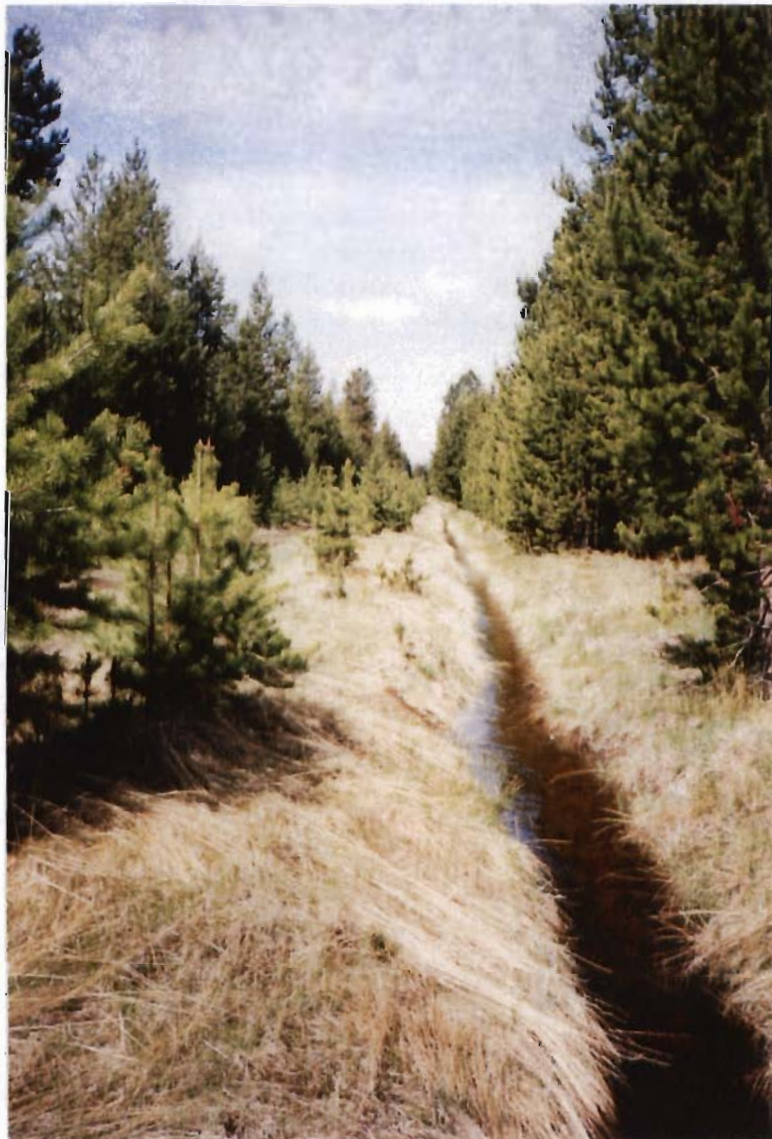
DIVERSION ditch to Foss going EAST 2003
