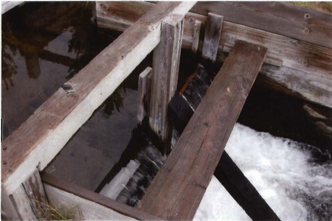
Main Canal Diversion For the Foss & Homestead 2003
