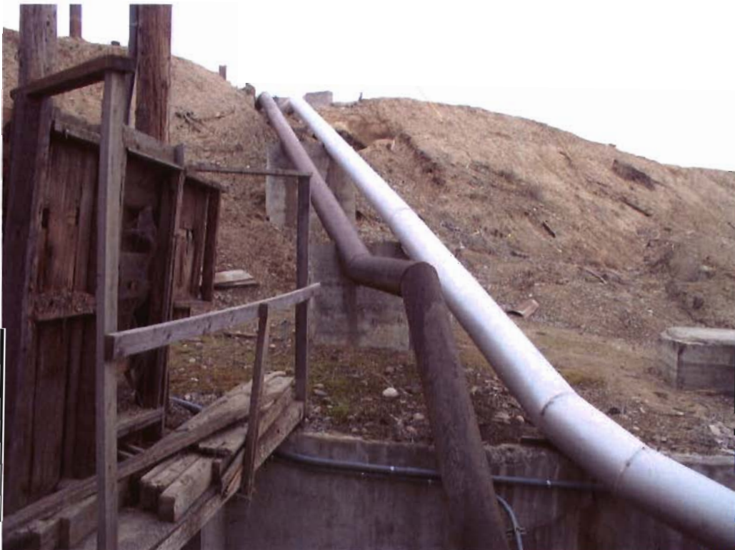
Existing Point of Diversion—Pipe Lines to Concrete Ditches
