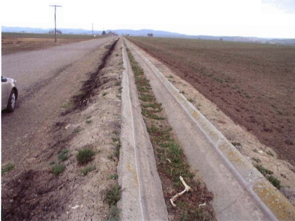
Concrete Ditch for Irrigating Fields
