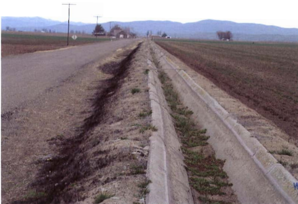
Concrete Ditch for Irrigating Fields
