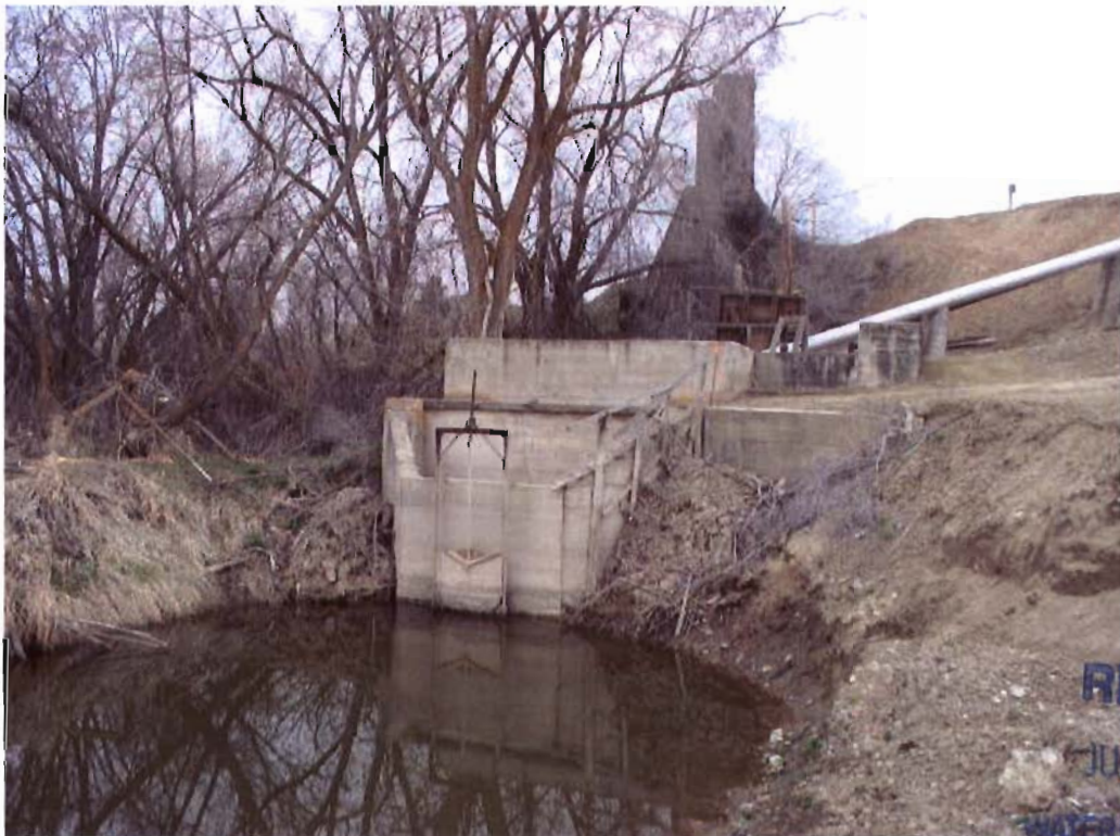
Existing Inlet Structure at Existing Point of Diversion
