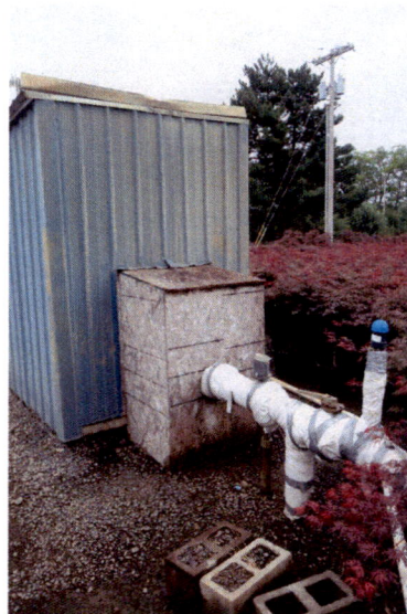
Well #1 with meter and filter in the background. Well #2, pump house, well box and meter.
