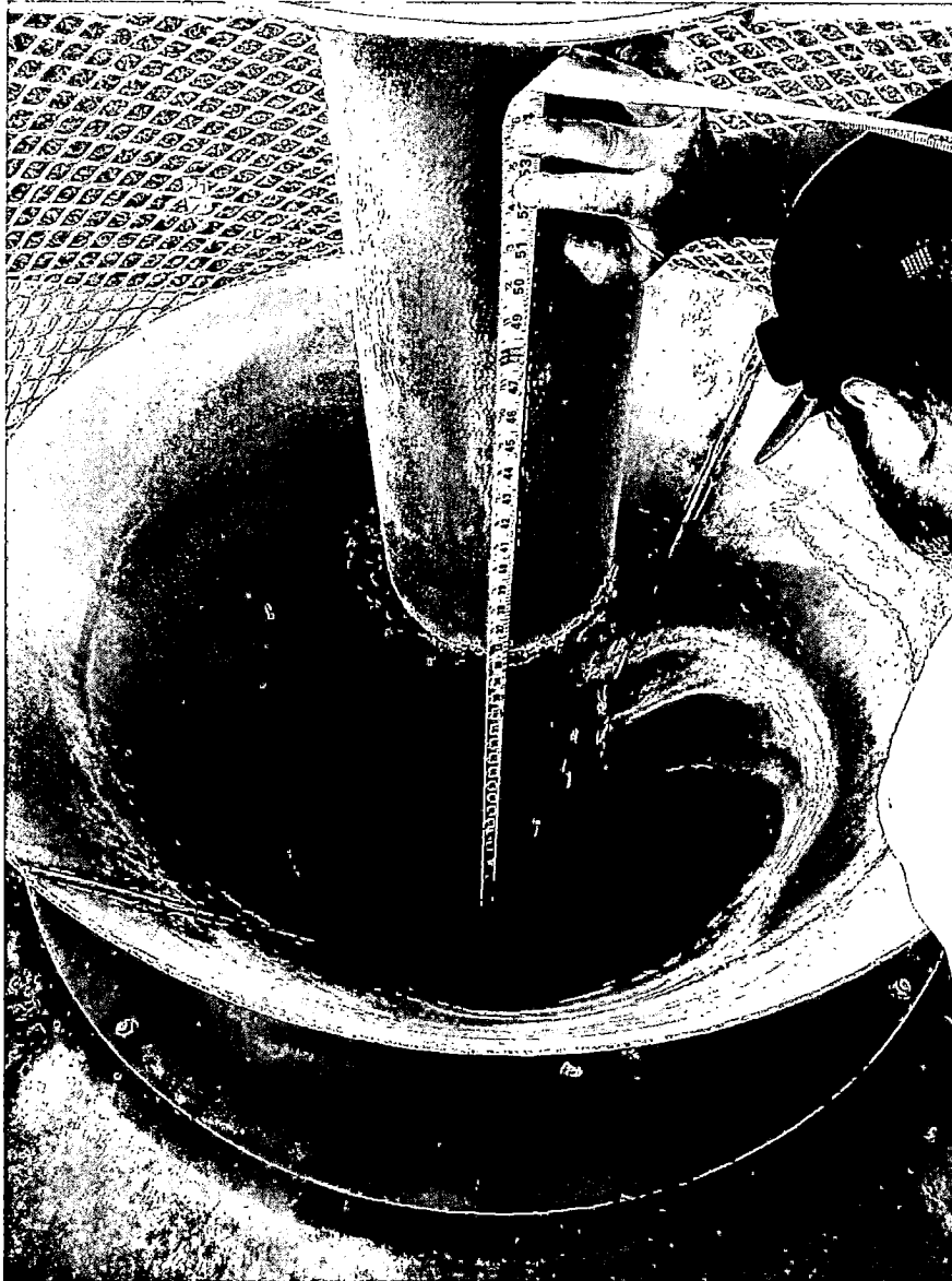
City Water Supplemental Water Pipe Discharge into Effluent Wet Well for Pumping of Recycled Water
