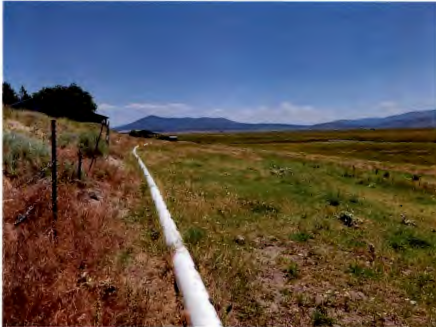
6" Mainline for Flooding
