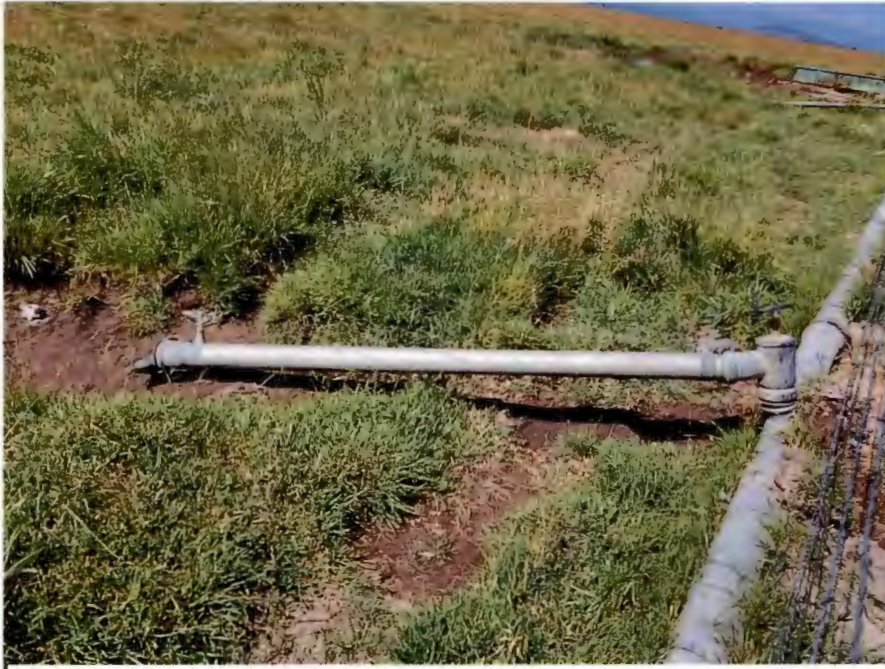
Mainline for Flooding
