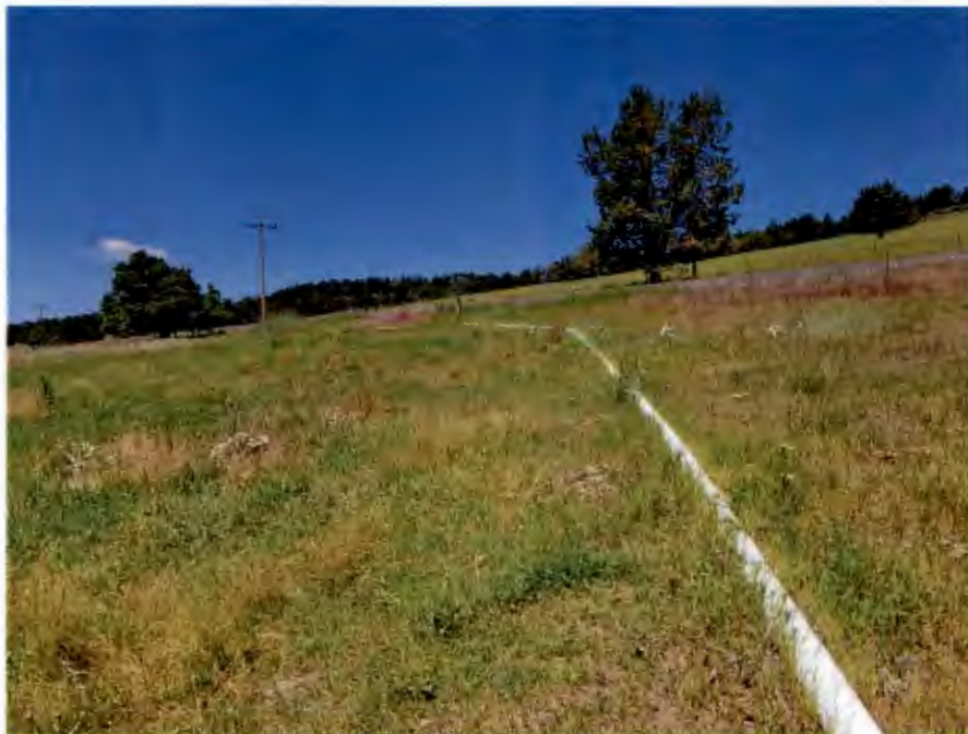
6" Mainline for Flooding
