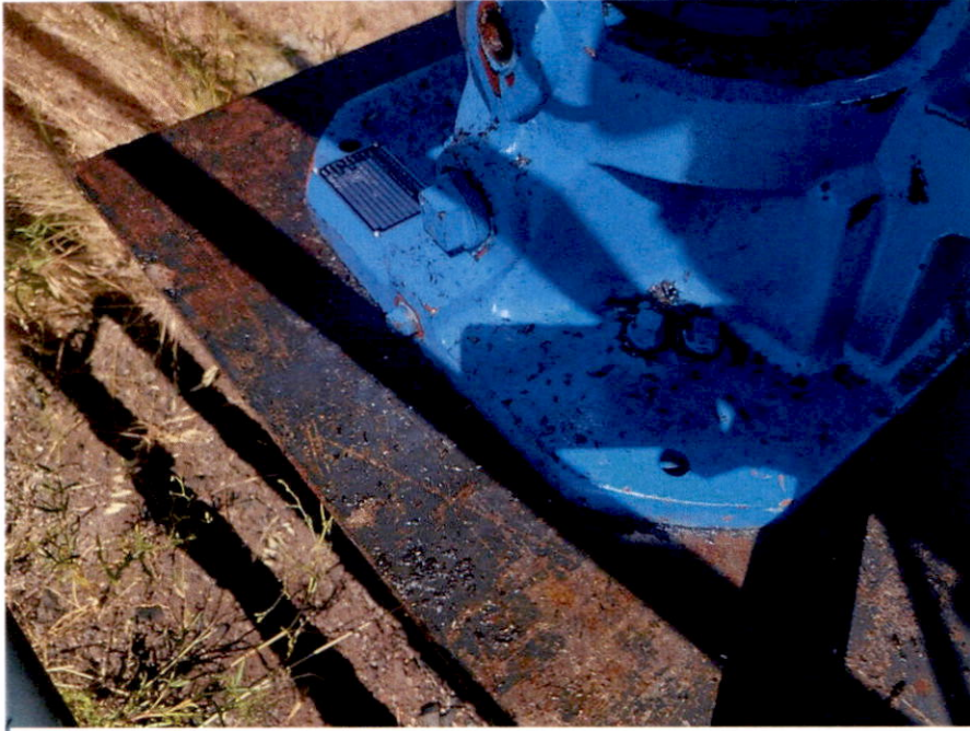
Well #5 Access Port
