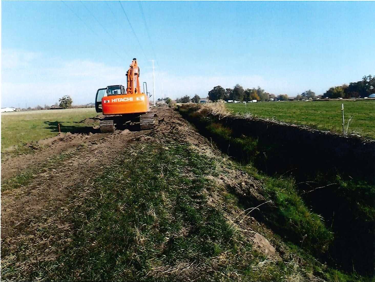
Figure 23. Photograph of the North Sunquist AR Site during Construction.
