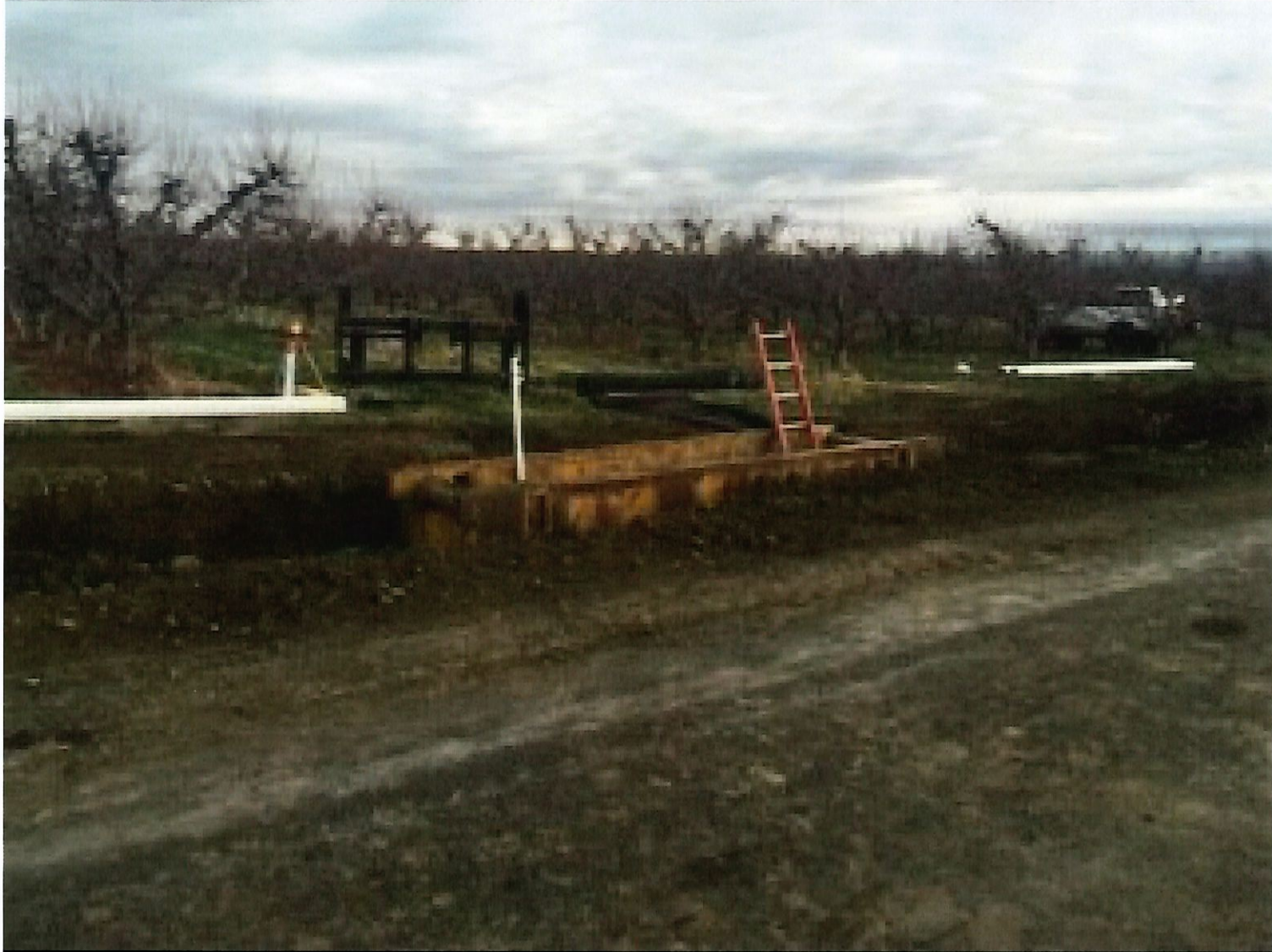
Figure 20. Photograph of the Miller Road AR Site during Construction.
