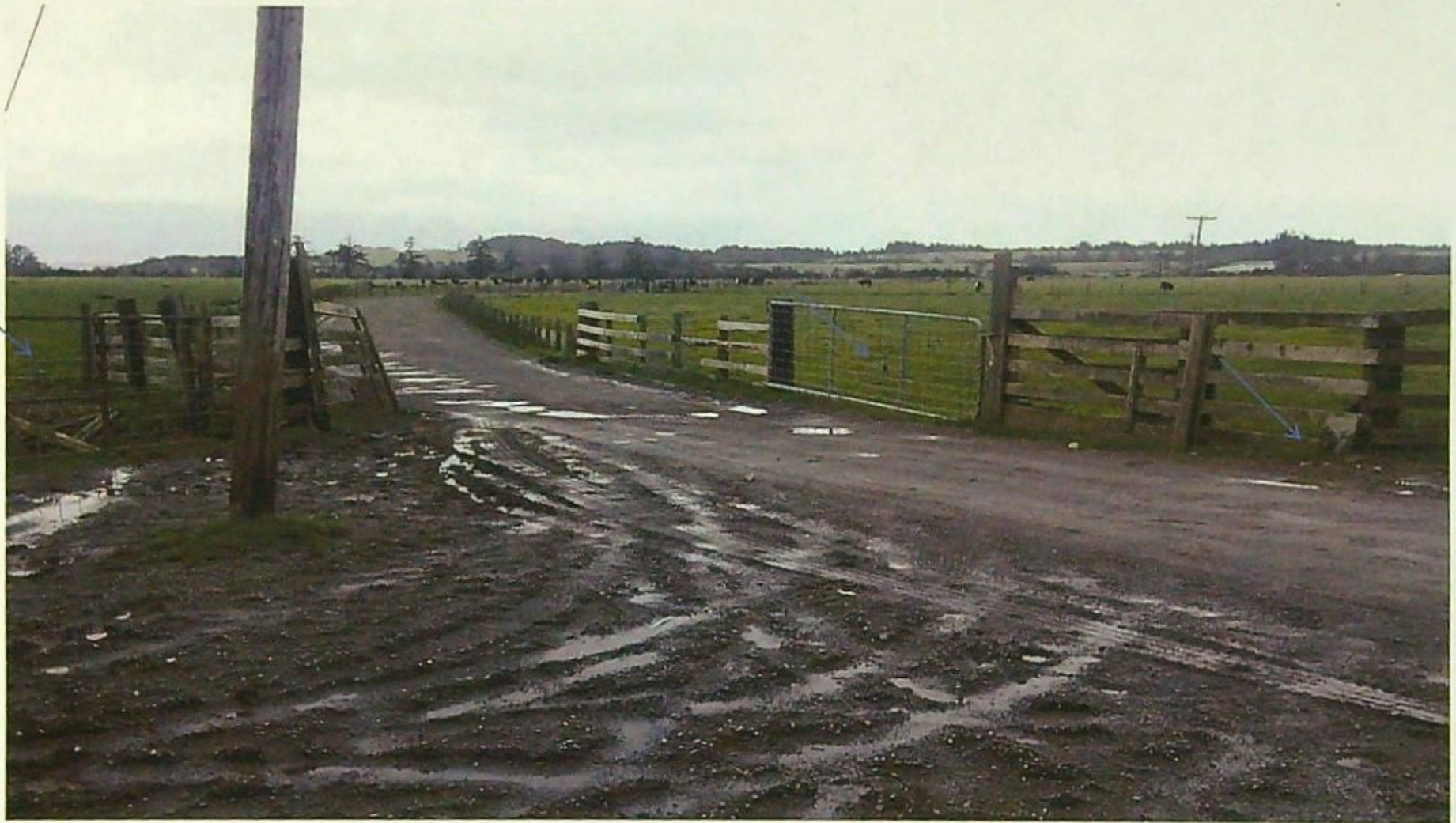
The access road to the Elk River, looking North, from the West side of the corral. The right hand arrow points to the pasture irrigation water meter. The other two arrows are irrigation valves, and the connecting points where the 2001 mainline installation connected to the previously existing mainlines.
