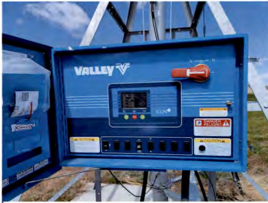
Pivot Control Panel
