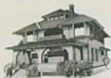
Historic Landmark Calhoun House ca. 1809
