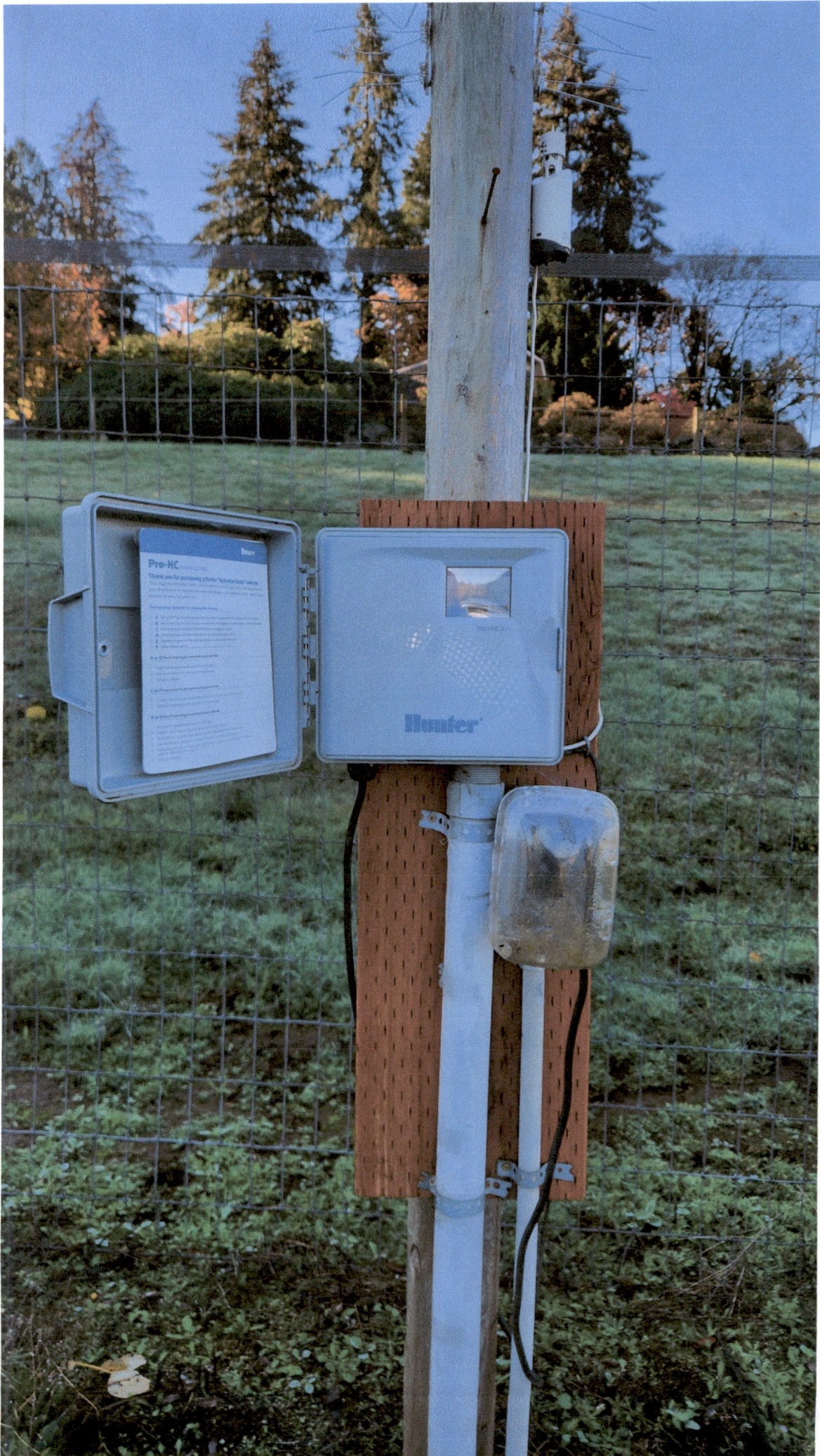
Jubitz COBU 11-6-24 Irrigation system time clock
