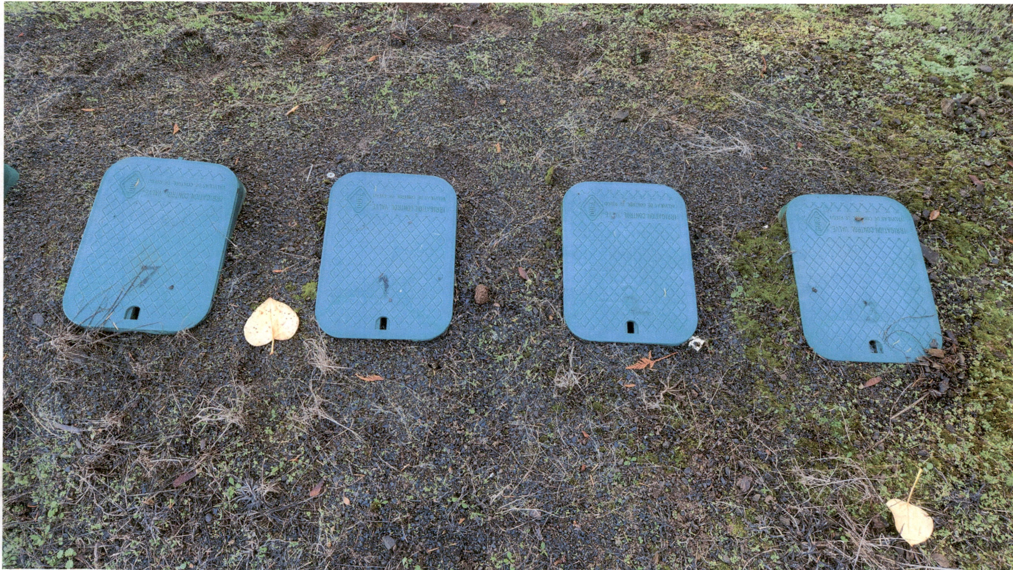
Jubitz COBU 11-6-24 Irrigation control valves (2" pipe inside)
