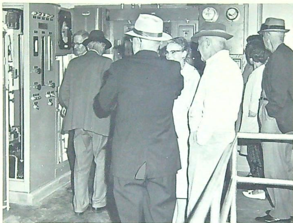
Control system of MicroFloc process, which doubled capacity of City of Silverton's water filtration plant, was center of interest during open house. City officials and employees and project engineers explained workings of new plant to townspeople.
