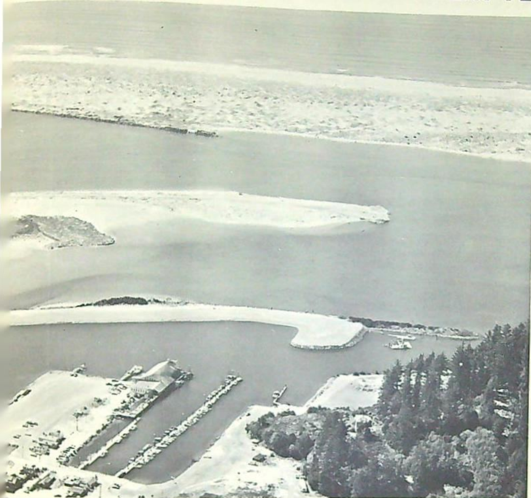
Breakwater at right center was first project in the development of Salmon Harbor at Winchester Bay. Tidal flats were dredged, carrying out master plan, to provide both boat basins and land for parking, roads, recreation and commercial areas.
