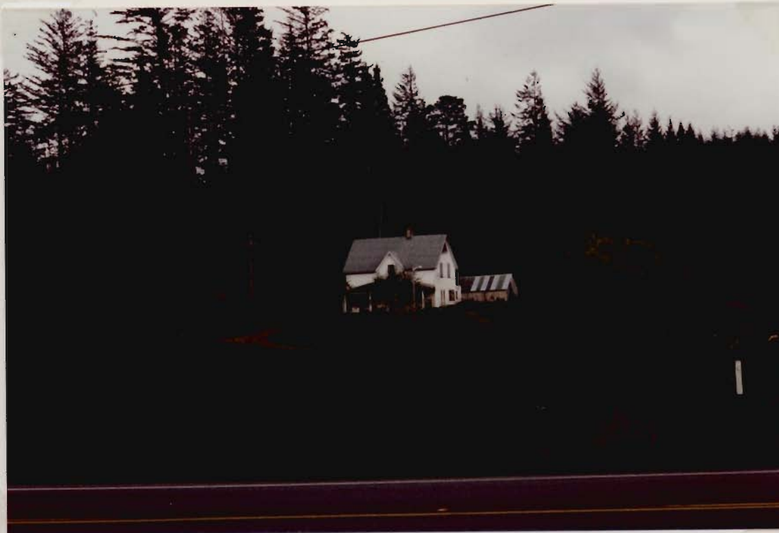
1992 PHOTO OF FARM HOUSE CONSTRUCTED IN 1900
