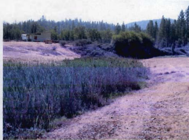
Area Between Roadfill and Embankment
