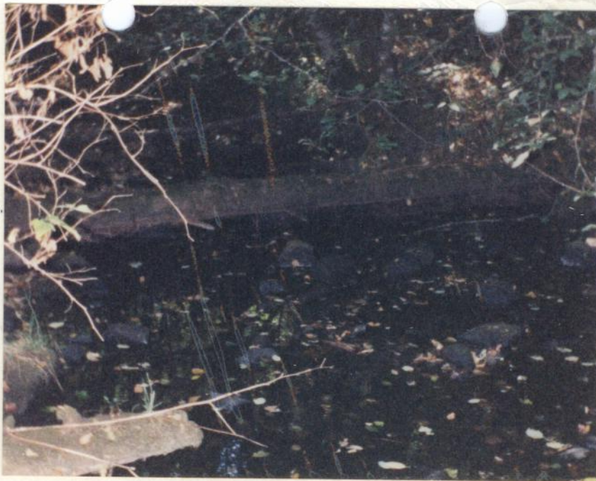
Footings of pre 1909 irrigation dam (looking upstream). Front sill reminent (left), rear sill log (back). Sill was preserved in gravel until 1950's and 60's when gravel gradually moved to fill 1945 in stream mill pond having it's own dam. Yet another dam upstream fed water to the 1945 mill boiler.
