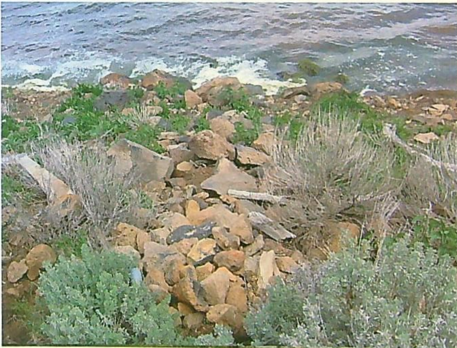
OUTLET VALVE STRUCTURE
