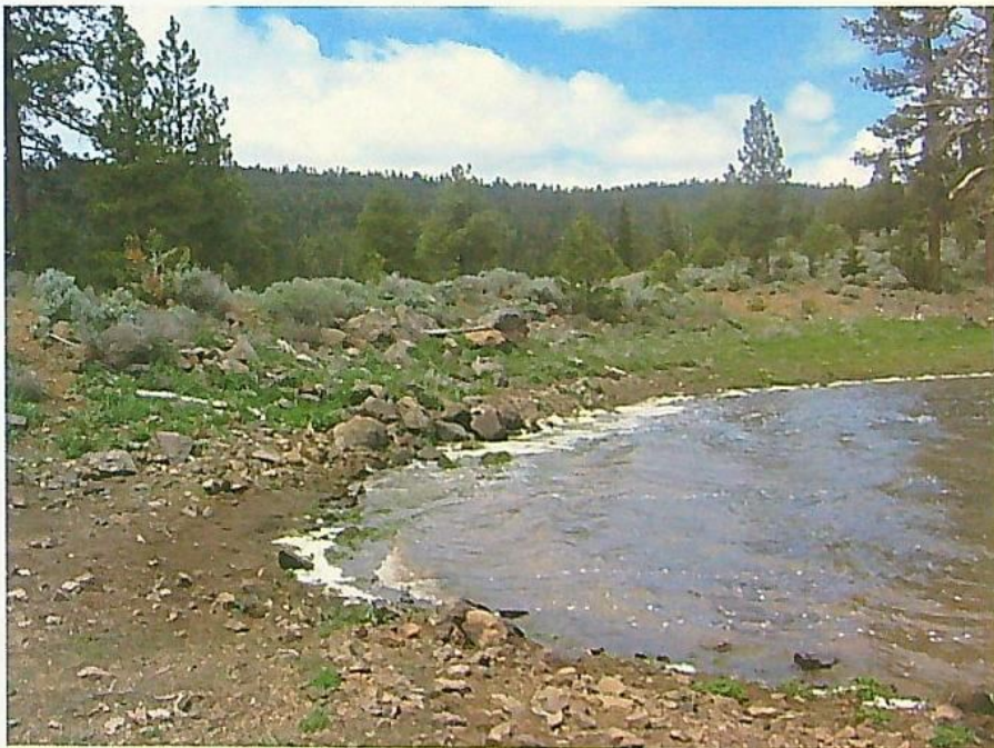
TAYLOR RESERVOIR DAM
