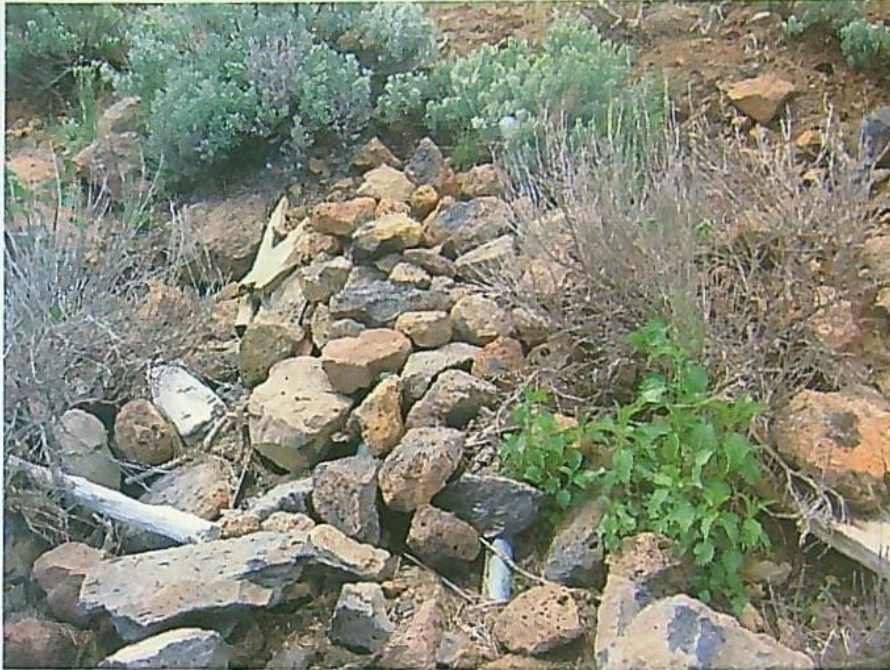
OUTLET VALVE STRUCTURE
