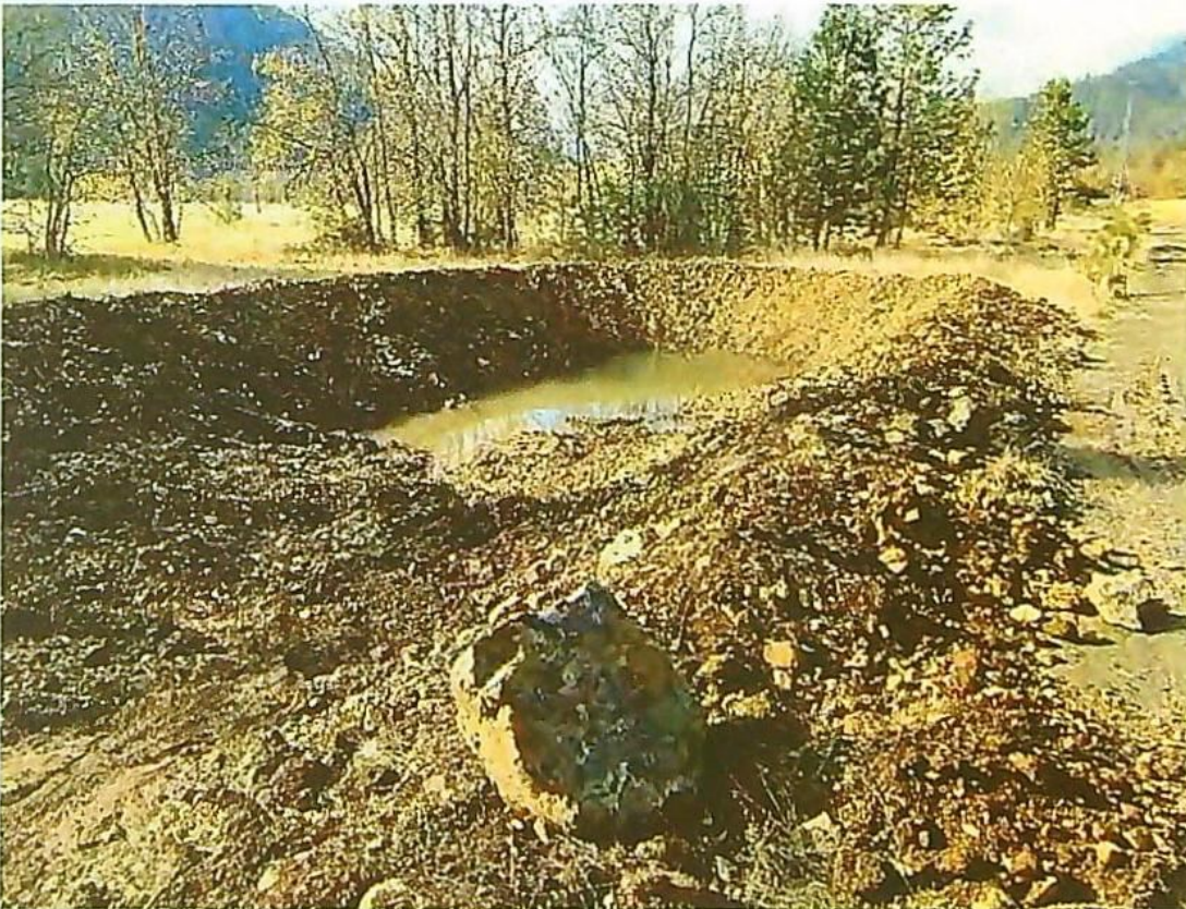
Photo 22 – Settling/Infiltration basin
