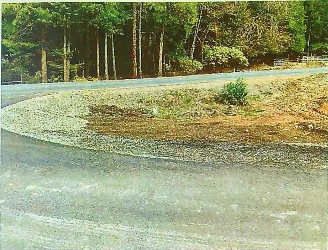
Photo 40 – Erosion at entrance- Needs erosion and sediment control
