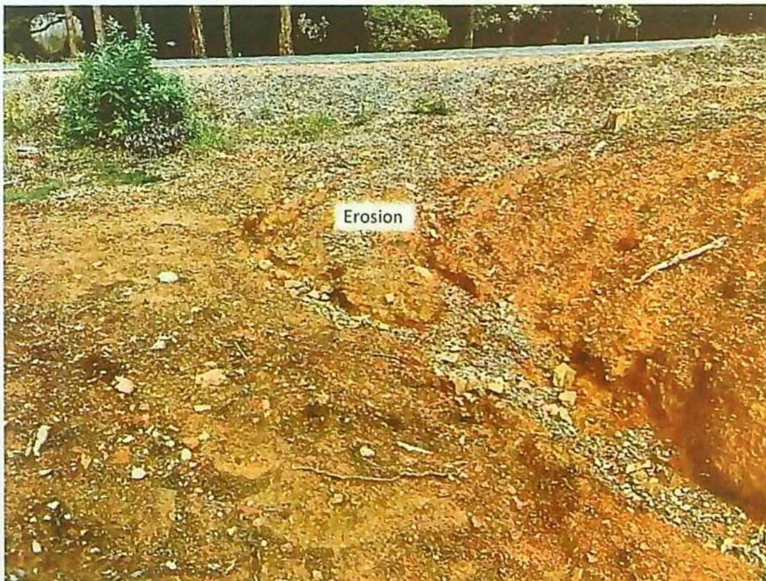
Photo 40 – Erosion at entrance- Needs erosion and sediment control
