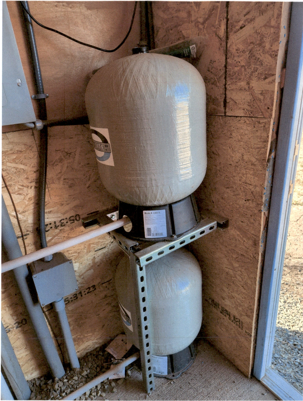
Tenbusch 9-13-24 COBU POA's 3 & 4 Pressure Tanks
