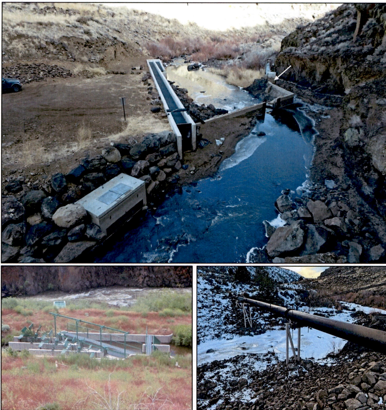
Figure 1. POD #1, the O'Keeffe Diversion on Deep Creek. Water is diverted through a headgate (white arrow, top photo), through a pipeline that crosses Deep Creek (lower right), into an open ditch with an ODFW rotary drum fish screen (lower left), and downstream to the Jones takeout (Figure 2).
