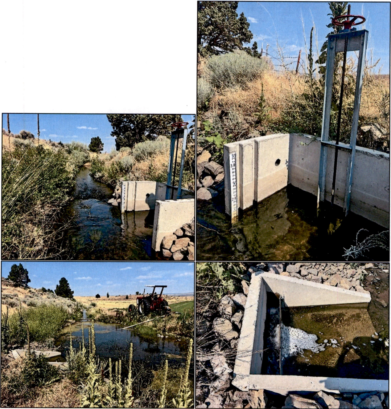
Figure 2. Jones takeout from O'Keeffe Ditch. Photos from August 1, 2024. Photos include the takeout from O'Keeffe Ditch (upper left), the staff plate in the takeout vault (upper right), the energy dissipation outlet vault at the downstream end of the HDPE pipeline (lower right), and the receiving pool in the Middle Ditch (lower right).
