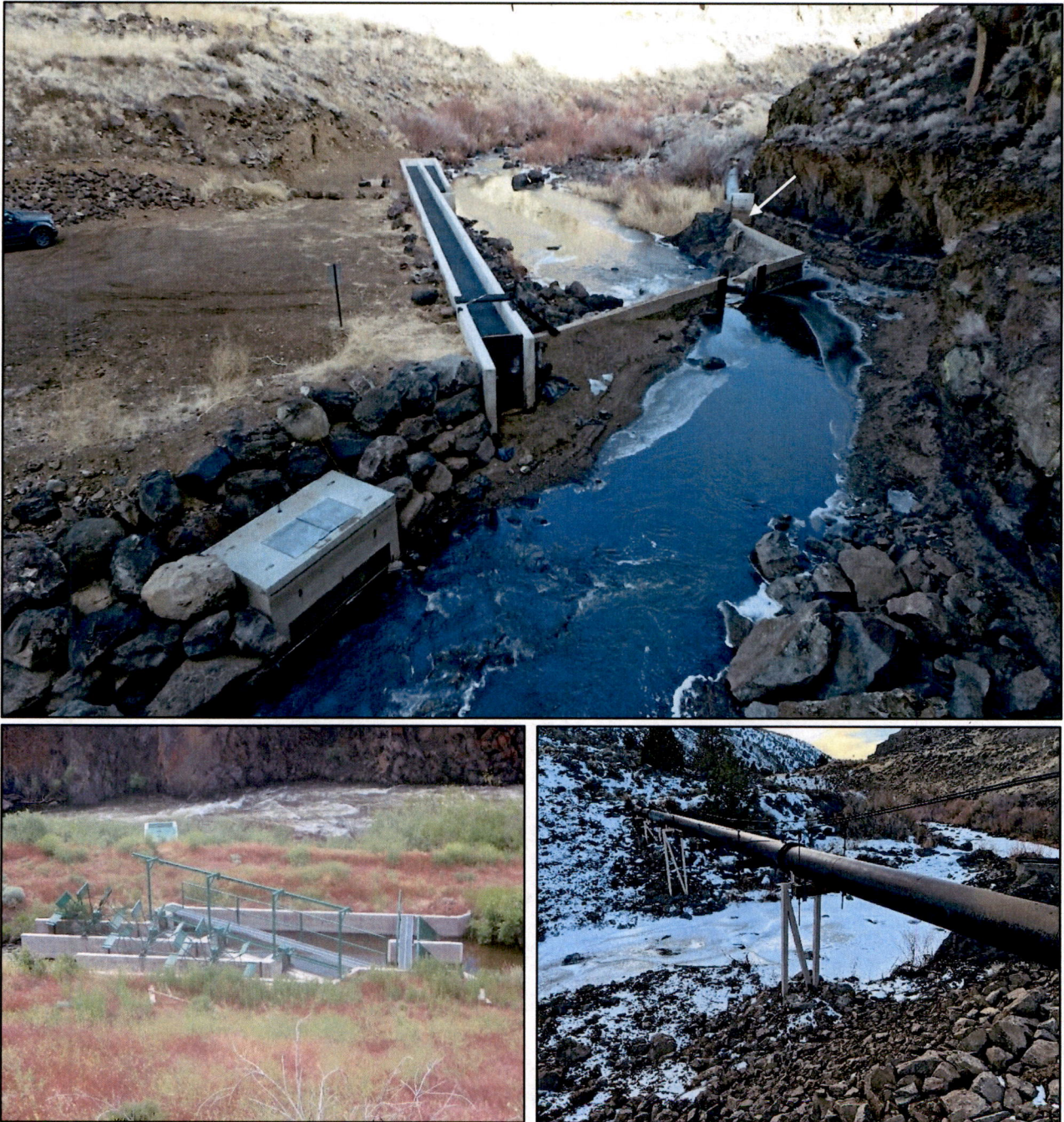
Figure 1. POD #1, the O'Keeffe Diversion on Deep Creek. Water is diverted through a headgate (white arrow, top photo), through a pipeline that crosses Deep Creek (lower right), into an open ditch with an ODFW rotary drum fish screen (lower left), and downstream to the Griener takeout (Figure 2).
