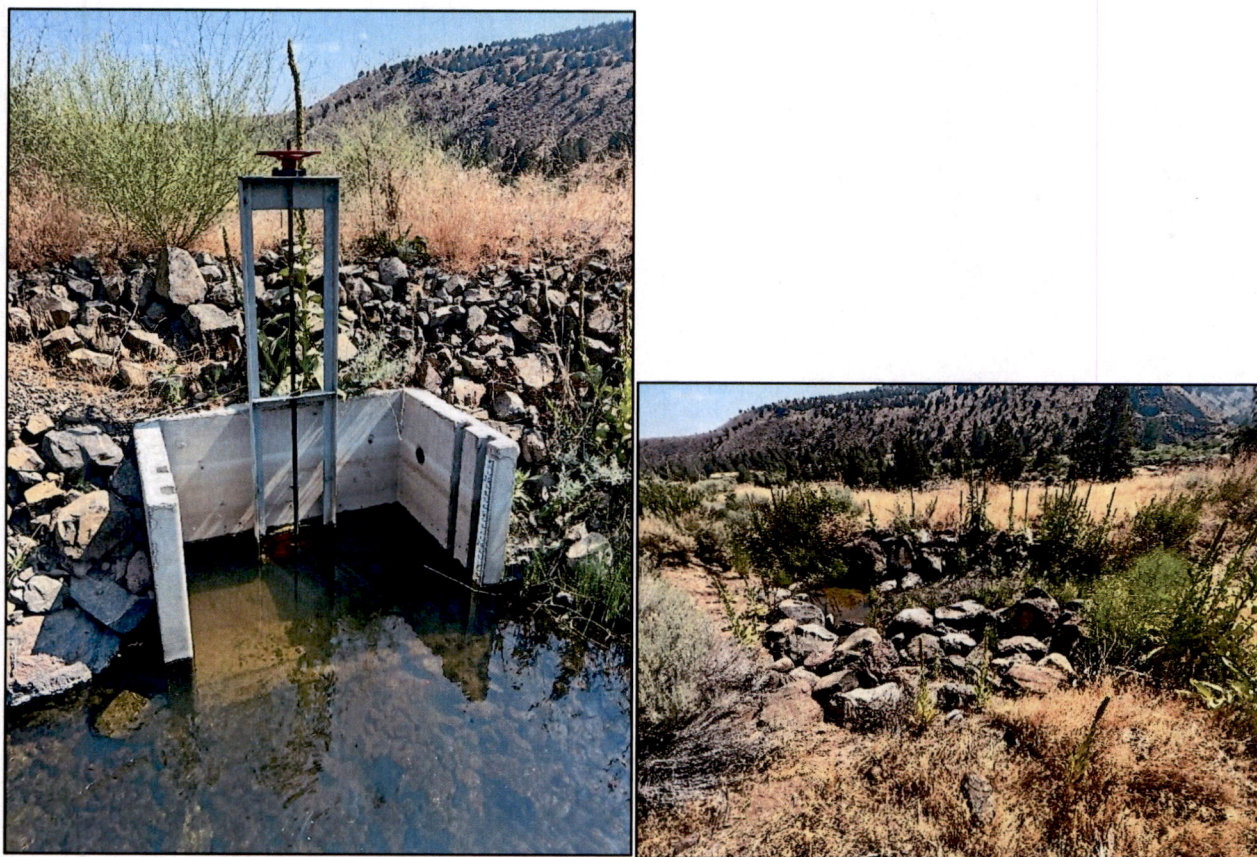
Figure 2. Griener takeout from O'Keeffe Ditch. Photos from August 1, 2024. Photos include the takeout from O'Keeffe Ditch (left). The staff plate is on the right wall of the concrete vault. The outlet pool in the Middle Ditch is located at the flume outlet (right)
