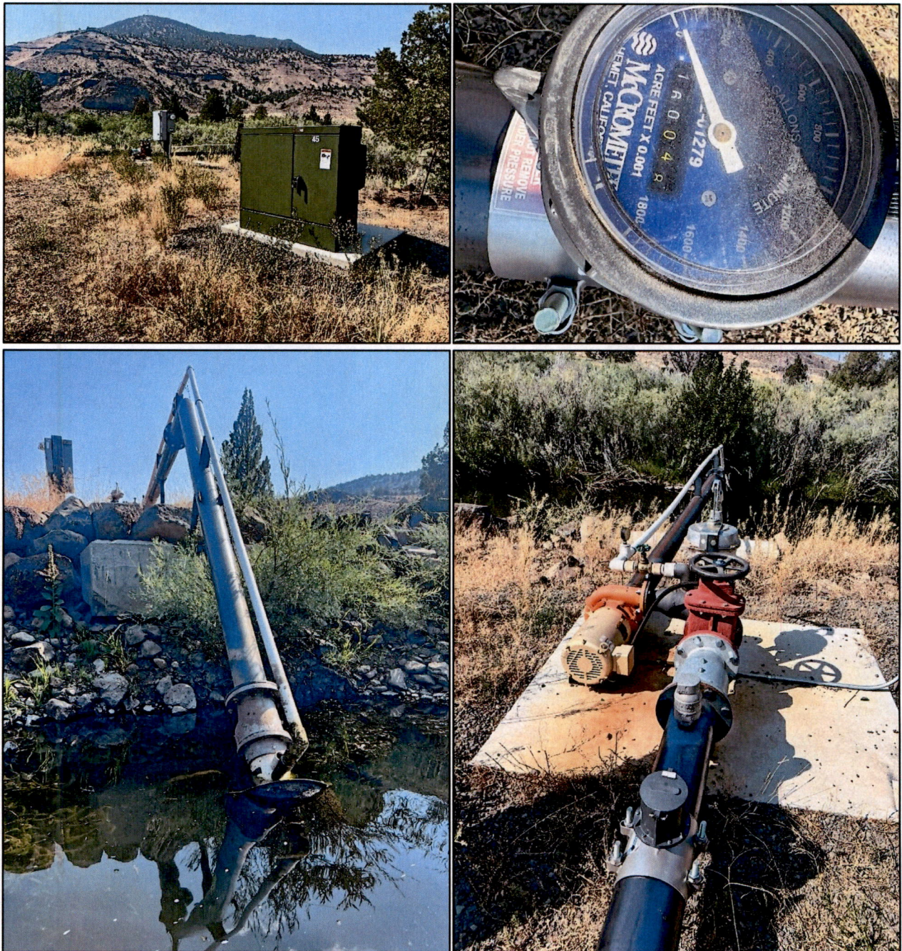
Figure 3. POD #4, the Griener pump station on Depe Creek. Photos from August 1, 2024. Photos include the transformer cabinet for the underground power lines (upper left), the McCrometer flow meter (upper right), the pump assembly (lower right), and the intake pipe with Sure-Flow self-cleaning strainer screen (lower left).
