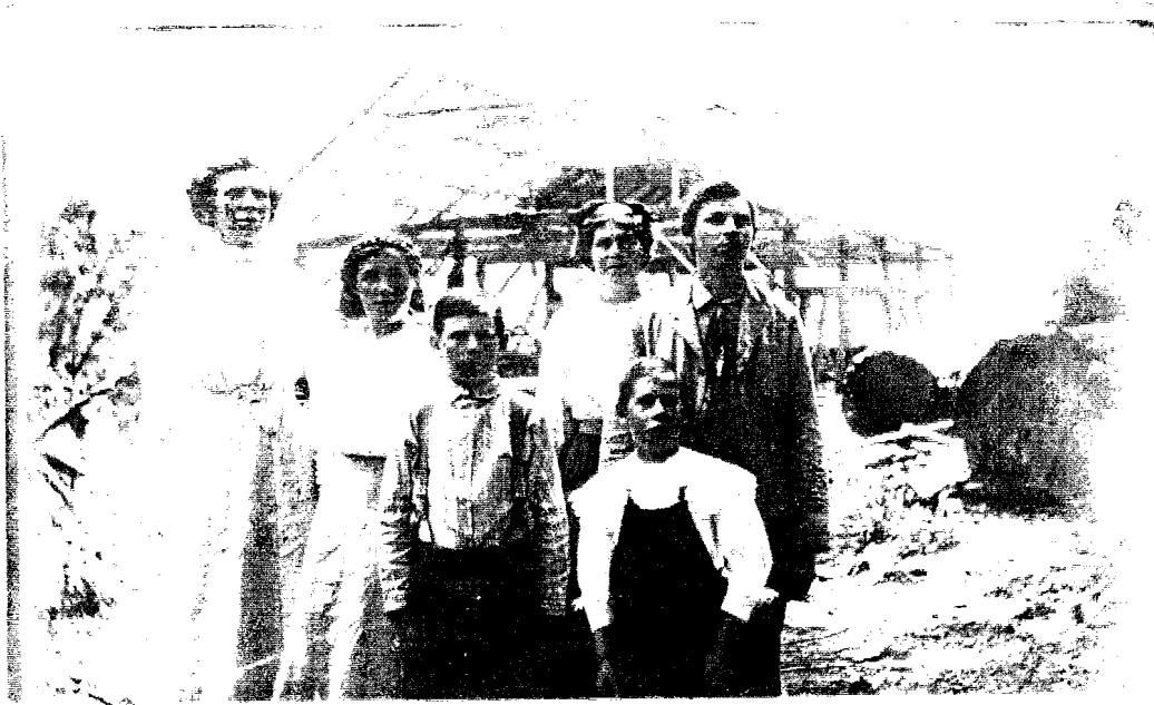
Construction of the Heller Sawmill located on Heller Homestead.
