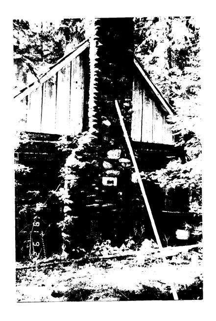
The old fireplace had no foundation and it was sinking into the ground. We tried to prop it up with a brace.
