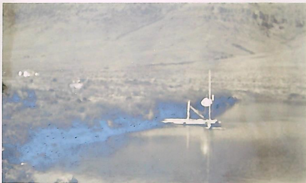
Outlet H.L. Dam - Sec. 30-35 \frac{1}{2} N - 32 \frac{1}{2} E.
