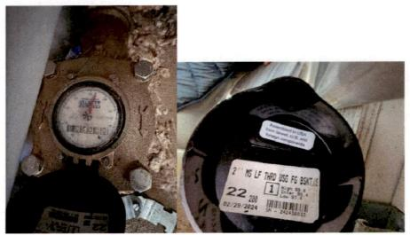
Totalizing flow meter conveys into a 3" diameter PVC irrigation main then to 1", 1.25", and 1.5" PVC laterals, then conveys to  $\frac{1}{2}$ " drip emitters to Place Of Use. No domestic use has been developed.
