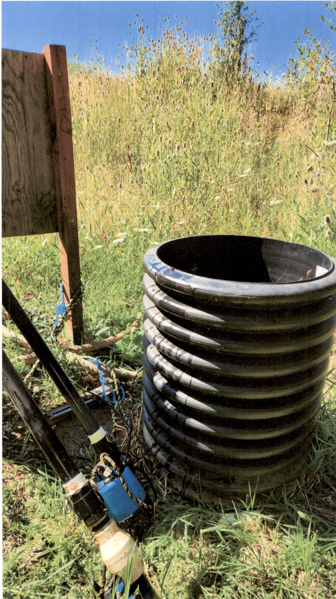
8-1-2025 Horton COBU 36" Culvert Pump Sump
