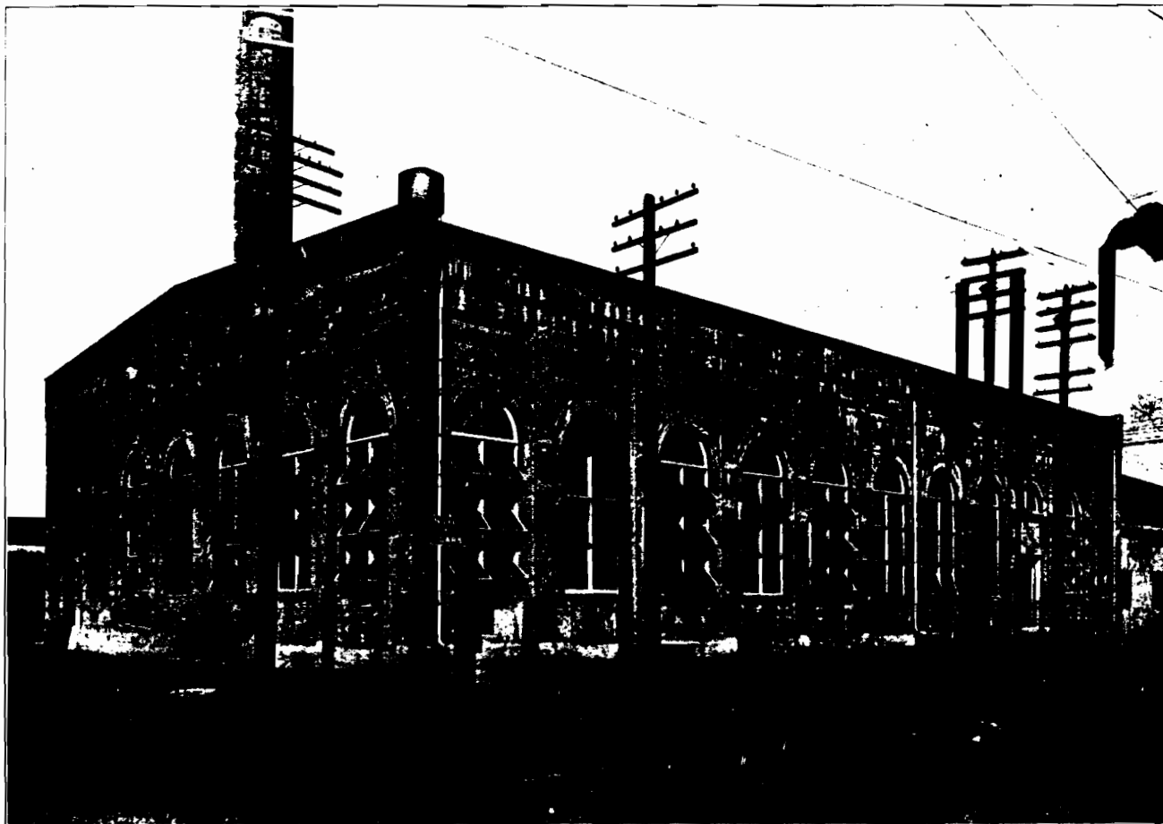
STATION E OF THE PORTLAND GENERAL ELECTRIC COMPANY, AT PORTLAND, OR.
