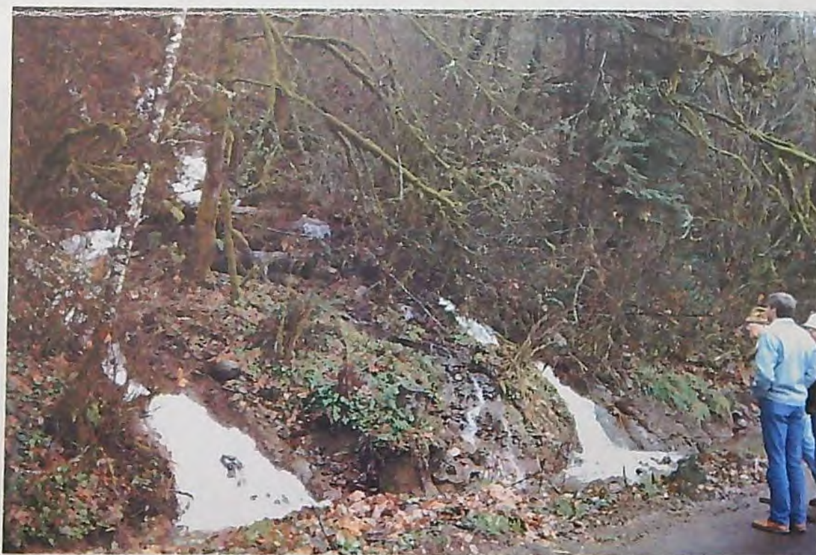
Photo No. 2 - Overland spill from Power Canal eroding channels in forested hillside, LaComb Hydroelectric Project, December 22, 1988.
