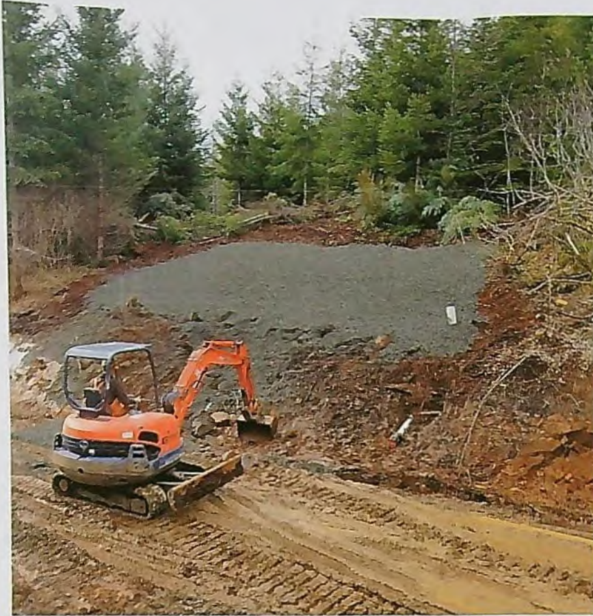
PHOTO 13 Finishing cover protection 02-15-2018
