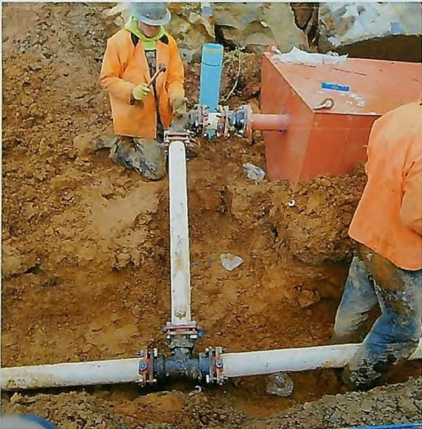
PHOTO 6 Spring Box and piping installation 01-12-2018
