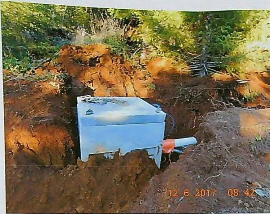
PHOTO 3 Installation of meter box
