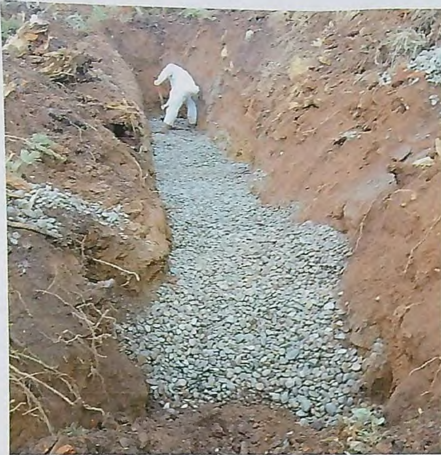
PHOTO 11 Backfilling spring intake 02-13-2018
