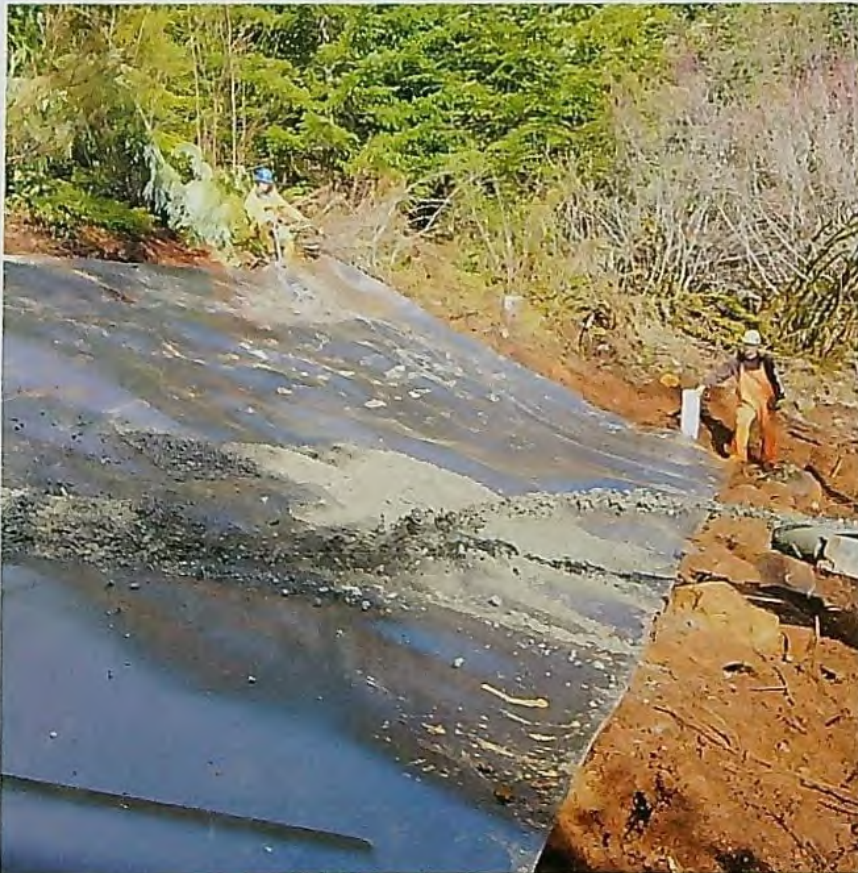
PHOTO 12 Installing cover protection 02-14-2018
