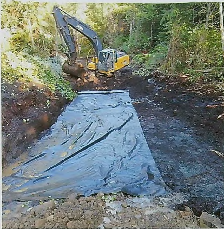
PHOTO 1 Construction of access road 10-14-2017
