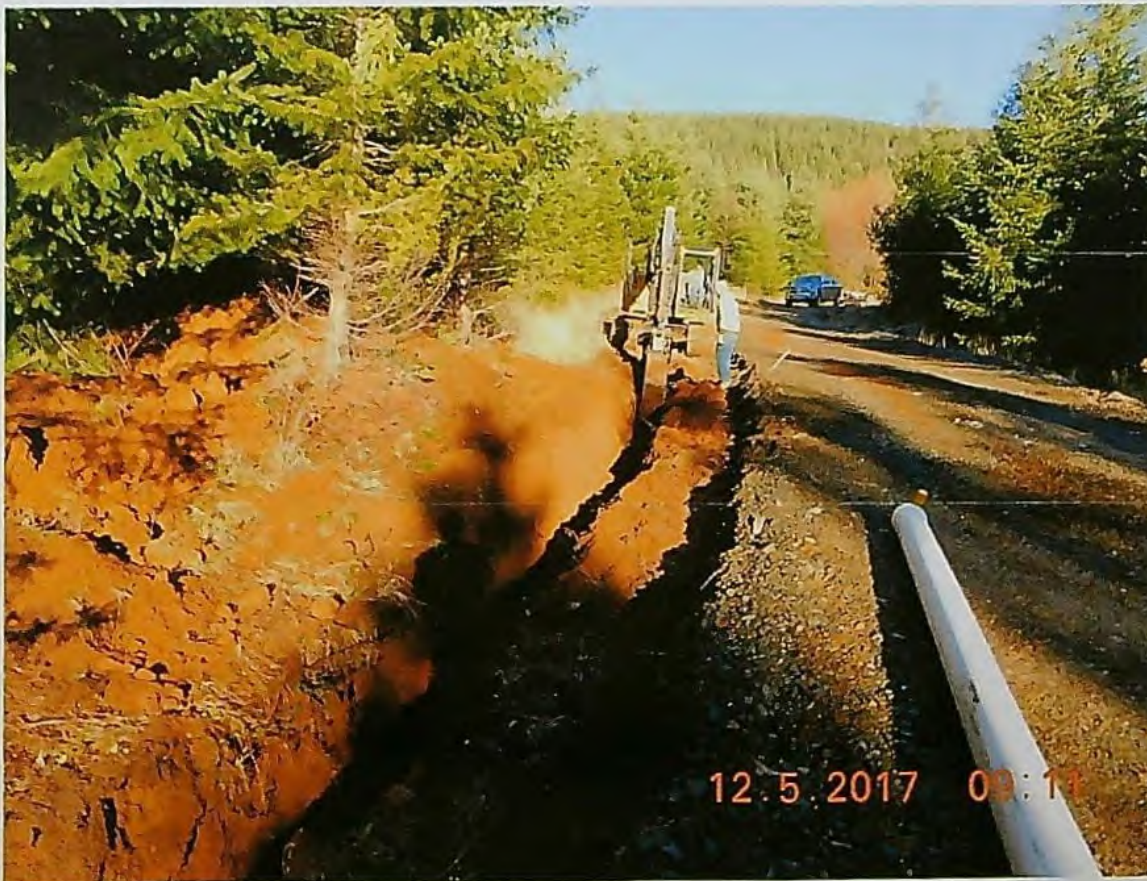
PHOTO 2 Installation of pipeline in access road
