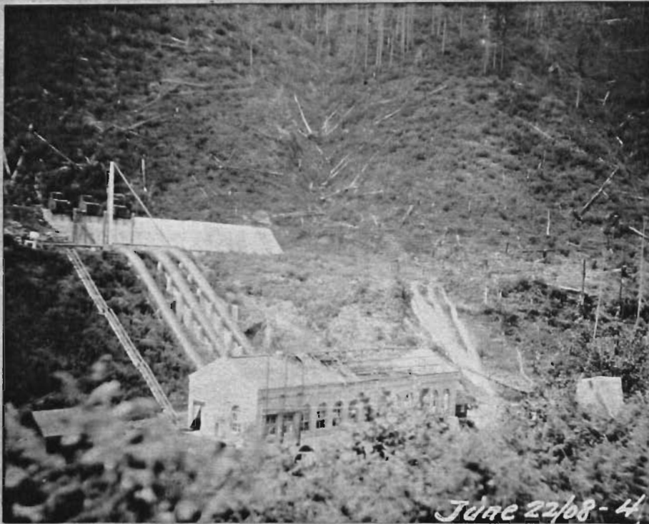
Cazadero - Exterior View Power House Day after Wreck.
