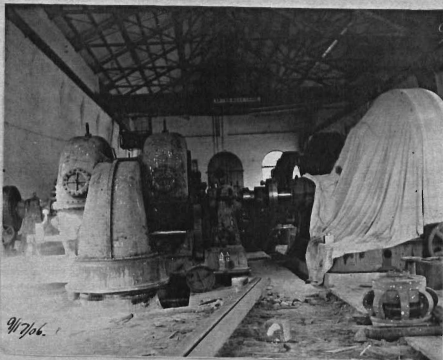
Cazadero - Power House Interior during Construction.
