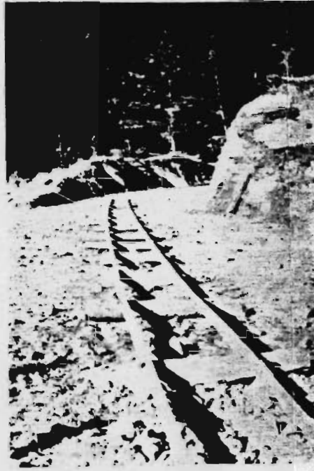
Wood tracks were used in building the Tiller-Trail road near Drew.
