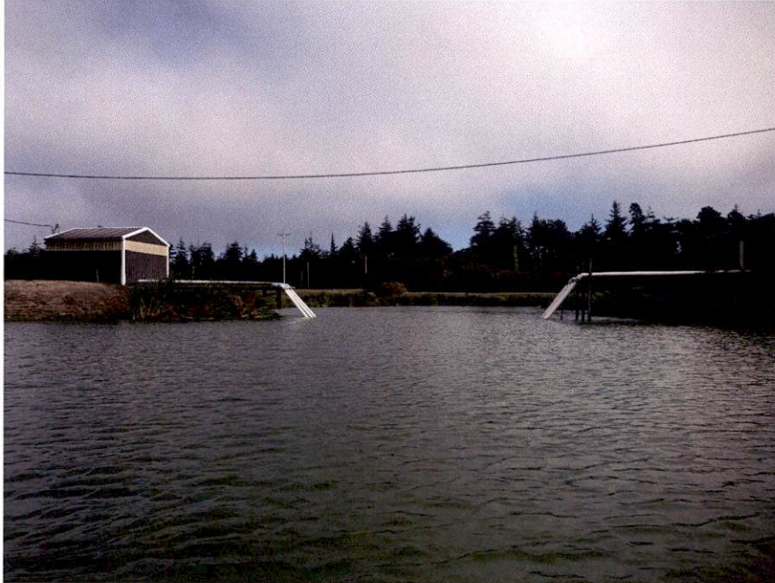
Reservoir 6 facing east, pump house on each side of the reservoir.
