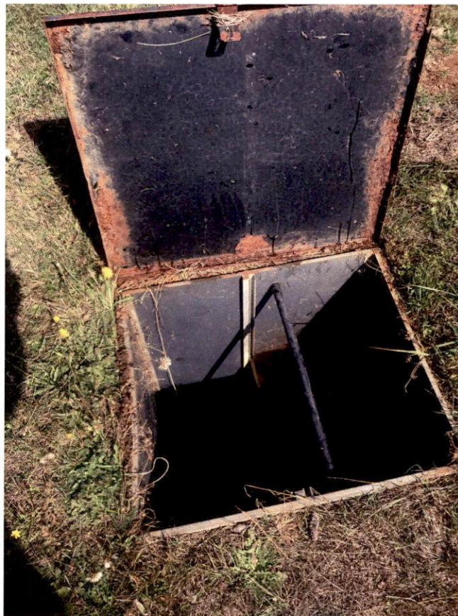
Reservoir 6, flashboard access for outlet pipe on northwest side of reservoir.
