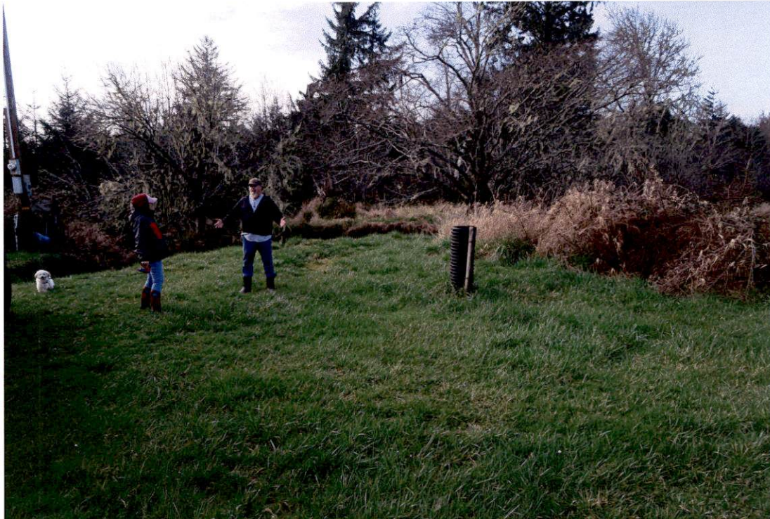
Two Mile Creek POD location, pipe standing up is to protect meter from high water. Electrical meter is visible on left side.
