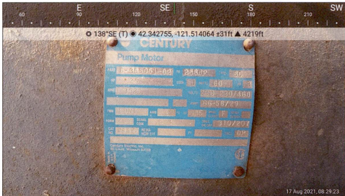
Figure 7: 25-hp booster nameplate at Well 2.
