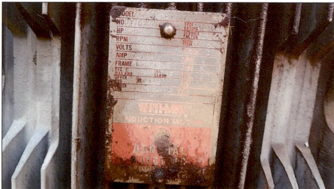
Figure 6: Well 2 motor nameplate (60-hp).
