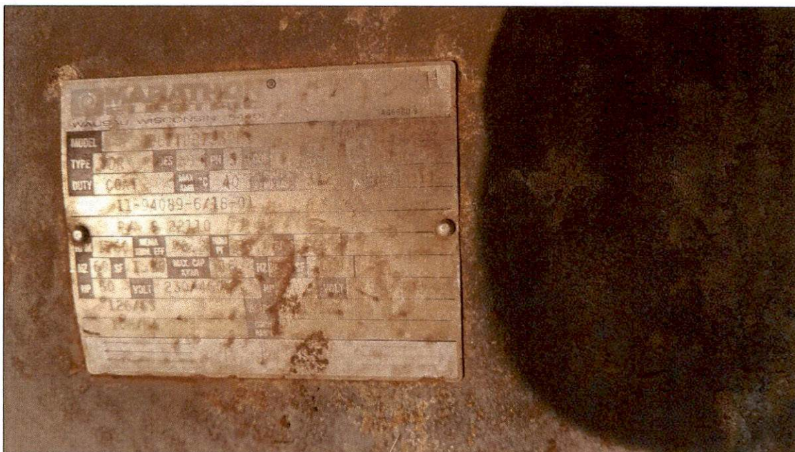
Figure 13: 50-hp booster motor nameplate at Well 3.
