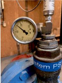
system, Well 9 at 1429gpm and 130psi.
