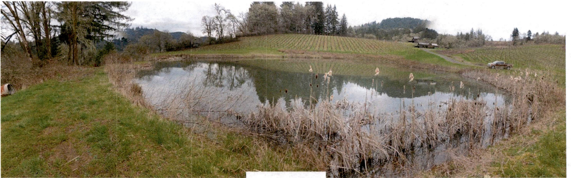
MARCH 19, 2025 Top of Dam, looking North (Panorama Composite)
