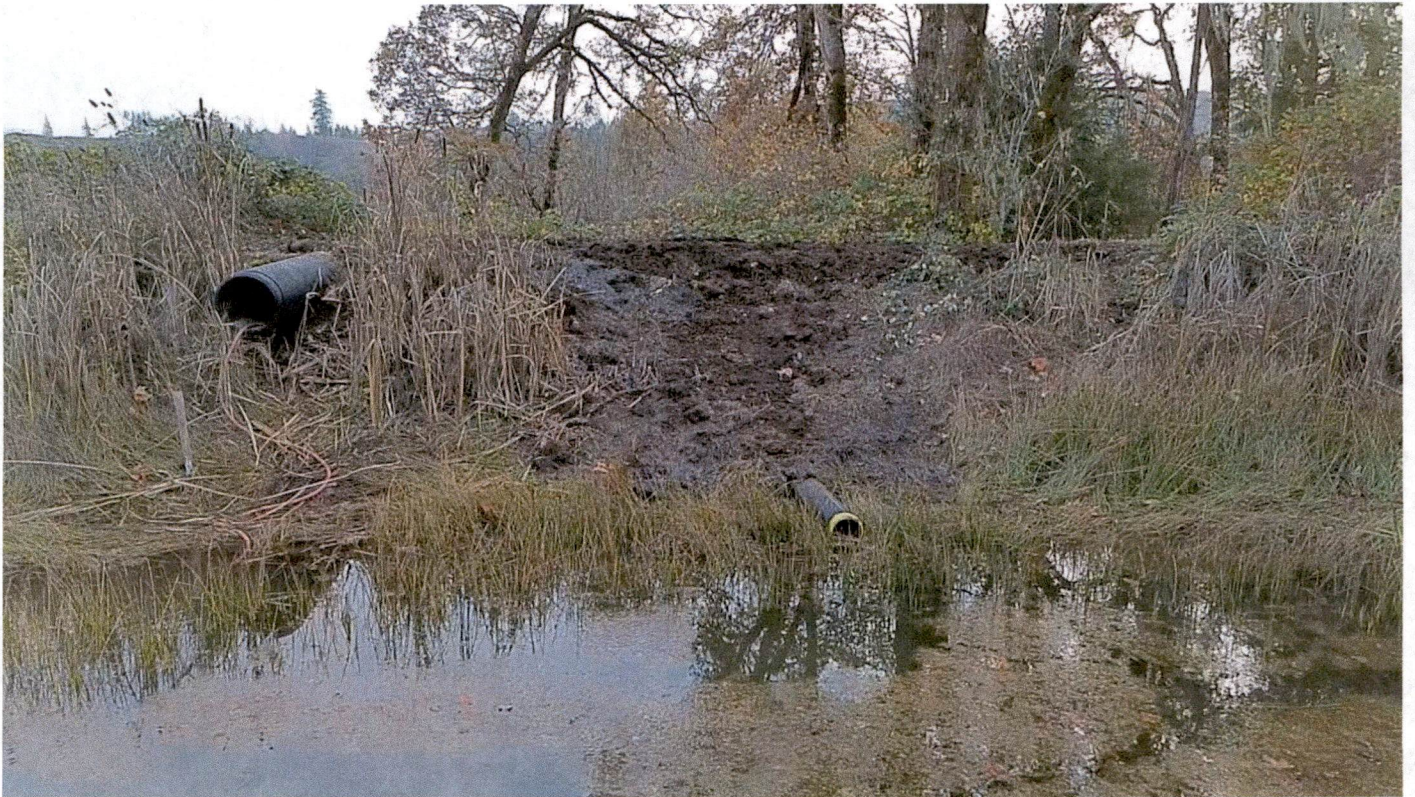
11-11-2025 Overflow modified to reduce storage to permitted 1.2 AF. Original overflow - upper left. Current, lowered, overflow - bottom right.
